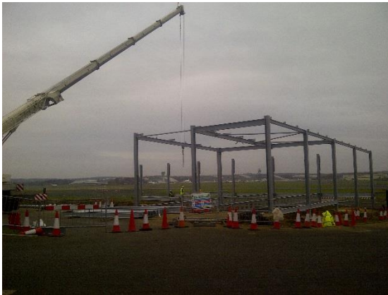
Construction of flexible building units at the site of Farnborough Airshow
