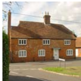
Old Basing. Many of the traditional buildings have first floor casement windows immediately beneath the eaves.
