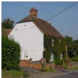
Highclere. Half-hipped roof with red clay tiles.
