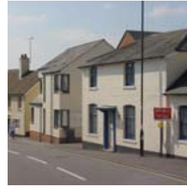
Whitchurch. Although the windows are not traditional in design, the scale of the building together with the colour and style of materials used ensure that it fits in with the general street scene.
