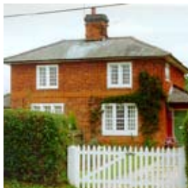
Stratfield Saye. Distinctive casement windows.
