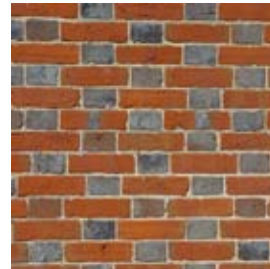
Tunworth. Brick pattering is characteristic of the area.
