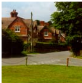
East End. Vertical clay tile hangings.
