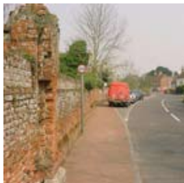
Old Basing. Brick boundary wall and buildings.
