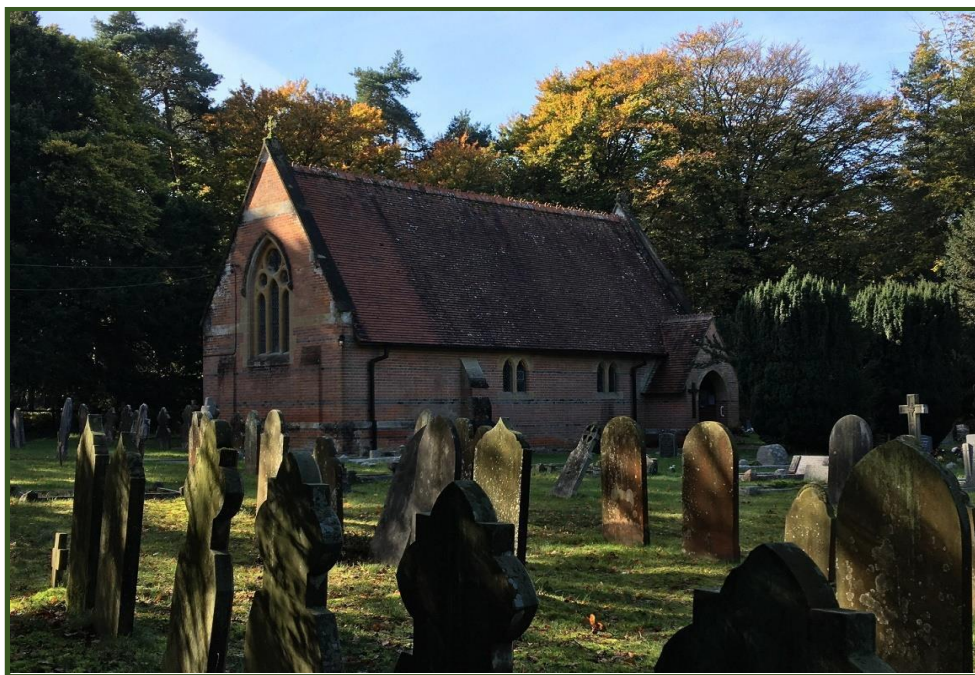
Figure 19 St. Peter's Church, Headley
