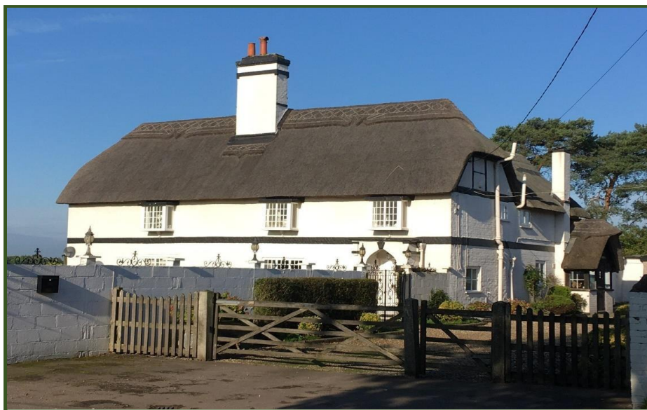
Figure 14 Ashford Hill Farmhouse (Listed Grade II)
