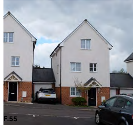
Figure 55: Three storey properties, Bishops Green
