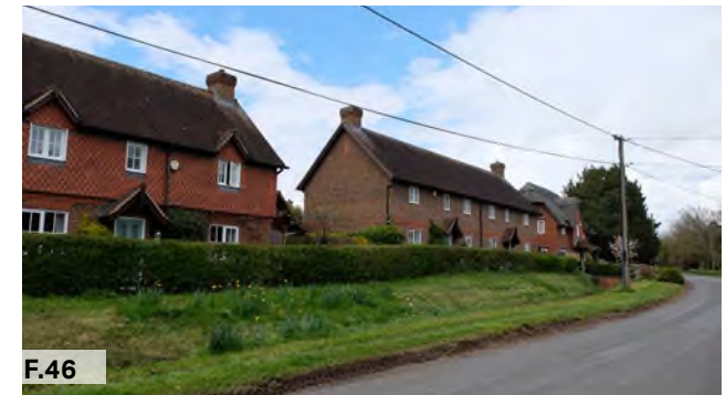
Figure 46: Brick cottages on Ecchinswell Road
