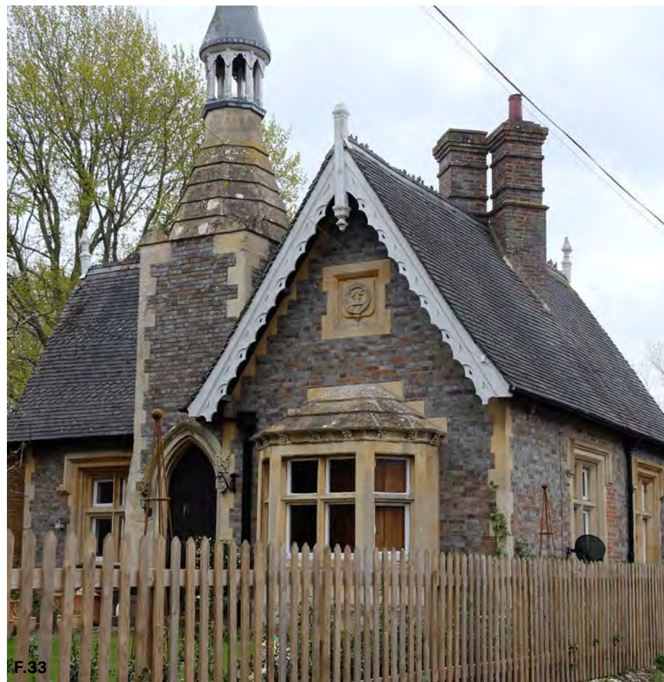
Figure 33: Grade II Ecchinswell School House
