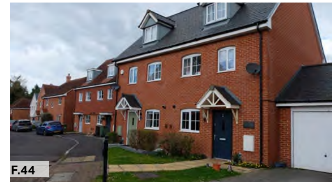
Figure 44: Semi Detached Housing in Ash Road, Bishops Green
