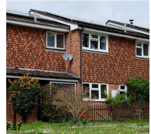
Figure 57: Two storey properties, Ecchinswell Green
