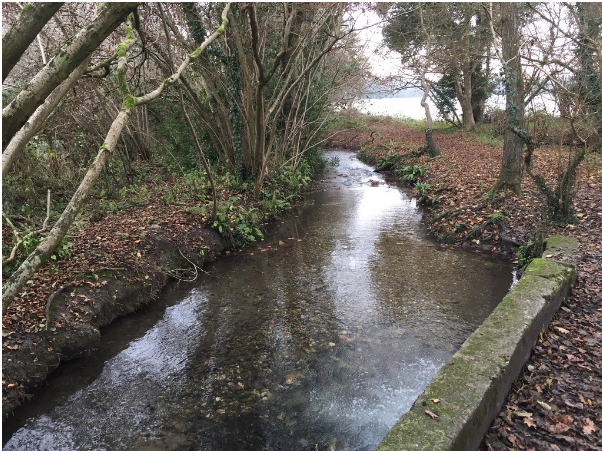
Ecchinswell Stream, near the pumping station
