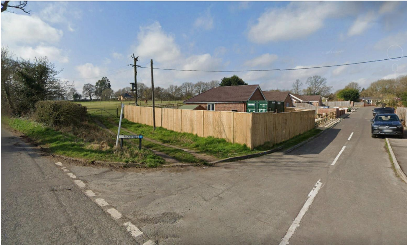
Fig. 7 Access off Rooksfield
