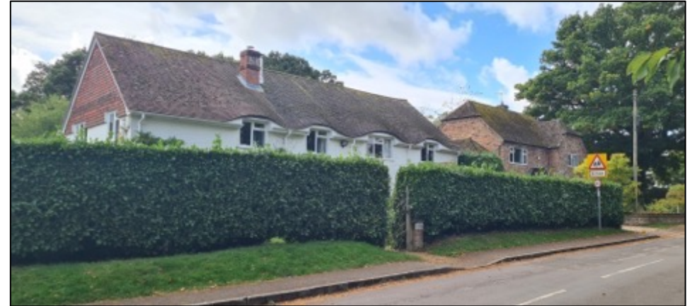
Unusual roofline of Old School Cottage
