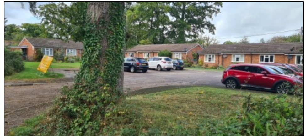
Low-density courtyard type development style at Elkington Close
