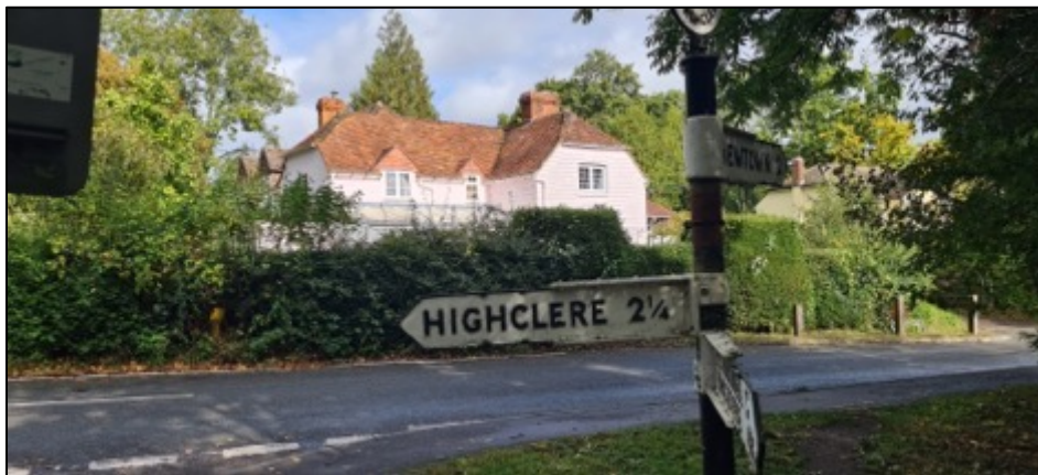
Locally Listed Building Grange Cottage
