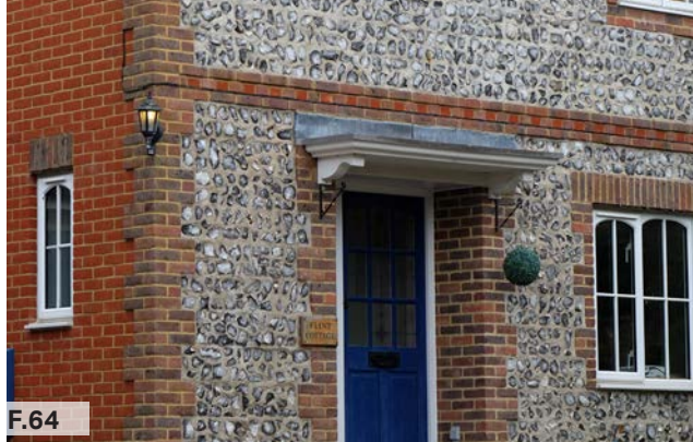
F.64 Figure 64: Red brick and flint walls, Ecchinswell Village Core
