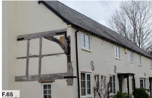
F.65 Figure 65: Pale render and timber framing, Ecchinswell Village
