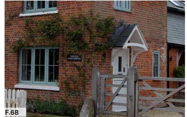
F.68 Figure 68: Door porch, Ecchinswell Village North
