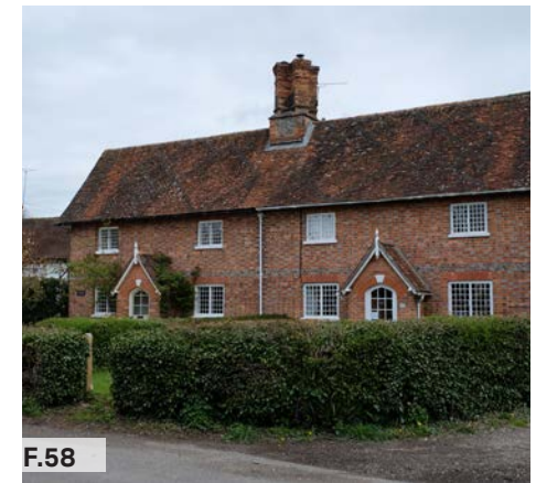
Figure 58: Two storey semi detached cottages, Ecchinswell Village North
