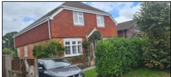
The use of tile-hung elevations in properties on Limes Avenue.
