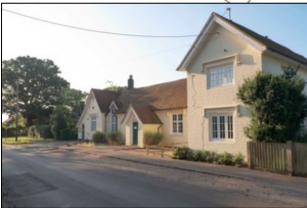
Locally listed Burghclere Primary School
