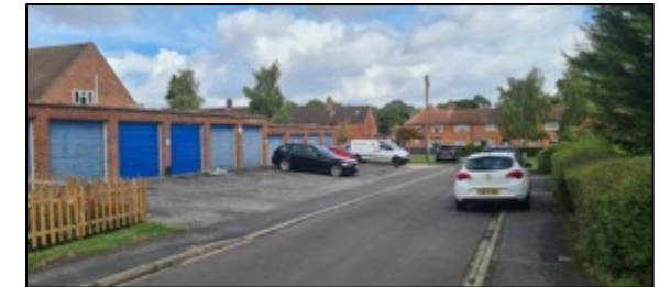
Row of garages providing some off-road parking
