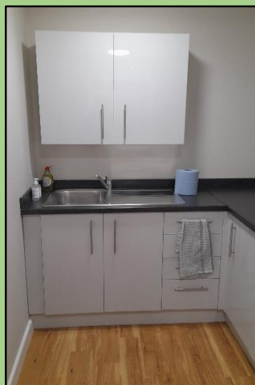
Osborne Room Improvements Viabes Community Centre, Basingstoke
