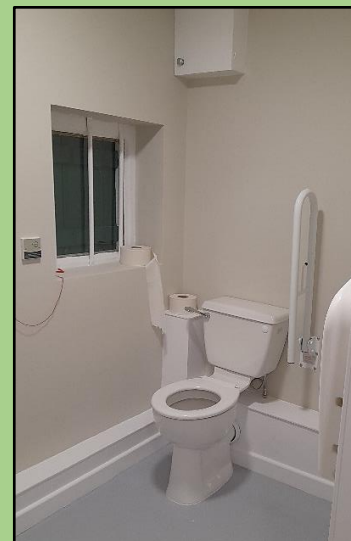
Toilet improvement works Viabes Community Centre, Basingstoke
