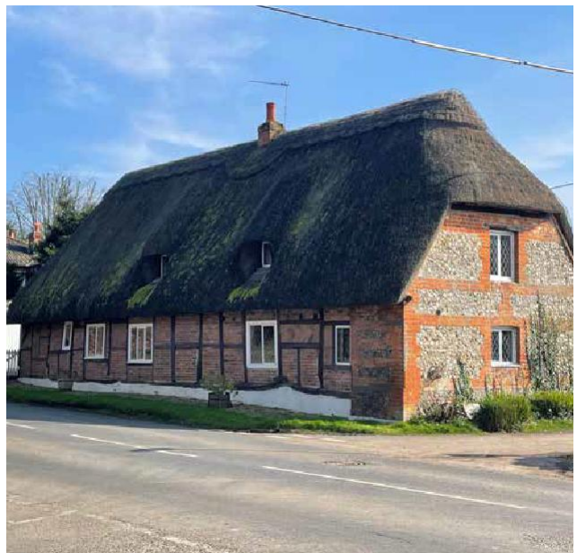
Figure 58: Listed thatched cottage using a range of traditional materials.
