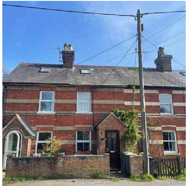
Figure 57: Historic red brick terraces on Kingsclere Road.
