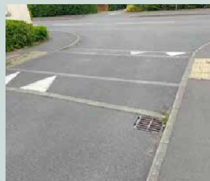
Raised pedestrian crossing
