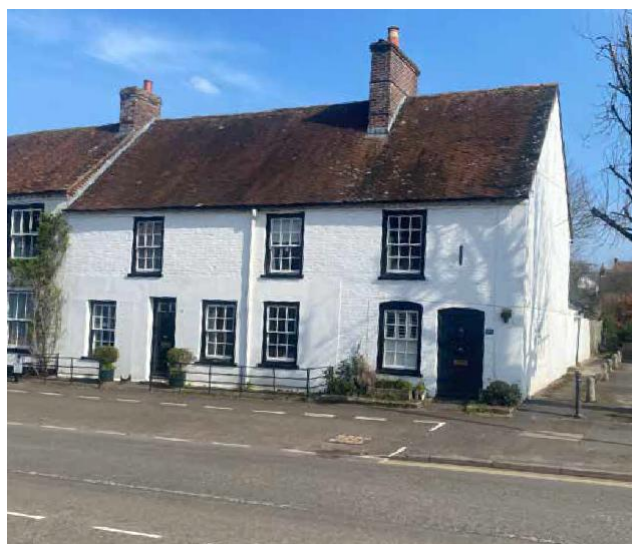
Figure 64: White render terraces on Winchester Street.
