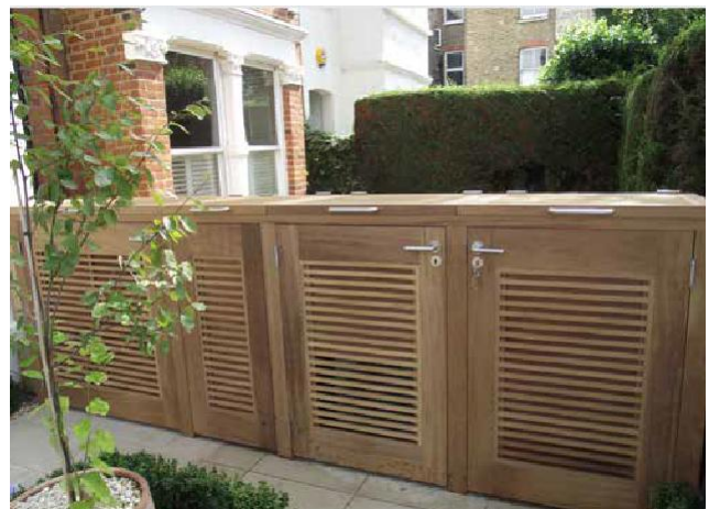
Figure 75: Examples of successful storage design solutions for accommodating bins at the front of buildings.
