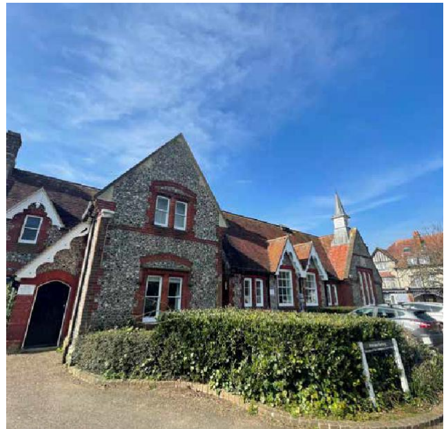
Figure 65: The Community Centre which uses flint and red brick.
