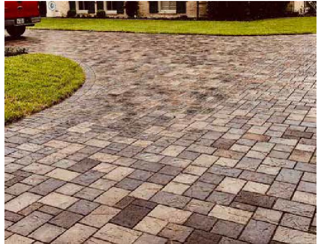
Figure 73: A good example of permeable paver (Source: https://www.paverconnection.com/testimonial/hedwig-village-permeable-driveway-and-patio-upgrade/ )
