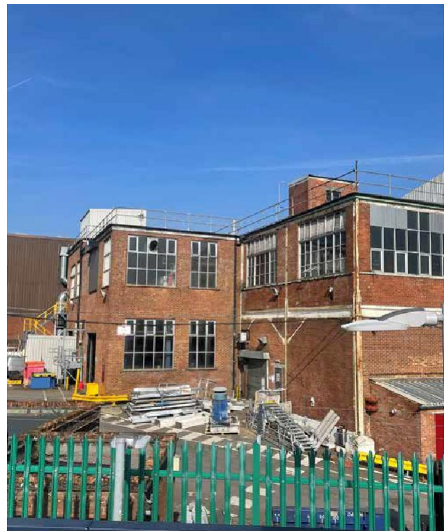
Figure 26: The disused Overton Paper Mill site.
