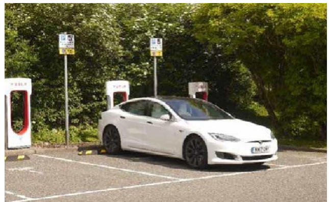
Figure 80: Example of electric vehicle charging points in a parking court.
