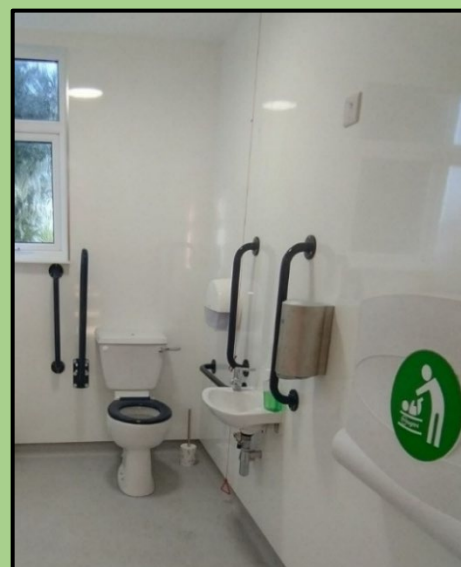
Improved Accessible Washroom
