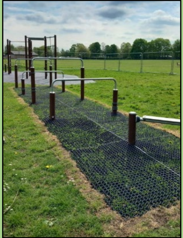
Improved Trim Trail Upper Sherborne Road, Norden
