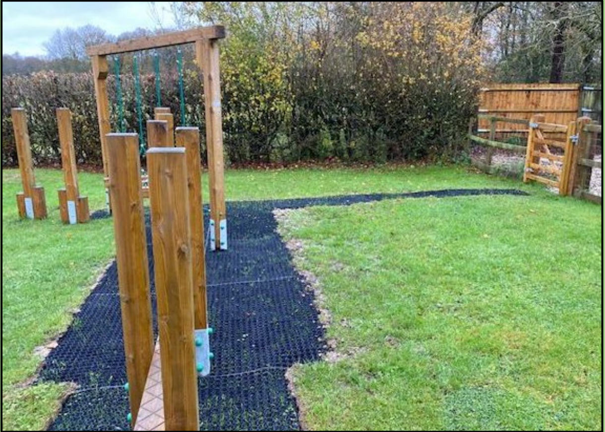
Grass reinforcement/matting to enable all season use Monk Sherborne Play Area, Monk Sherborne.
