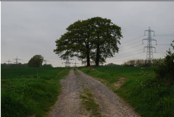
Photo 5: View west along farm track west of centre of site, towards electrical sub-station at Bramley Frith Wood.
