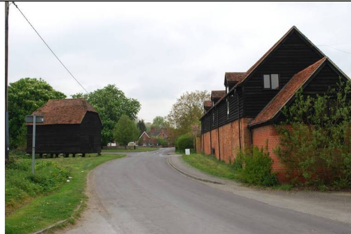
Photo 8: View south along Minchens lane from entrance to recreation ground adjacent to site. Listed structure visible on left.
