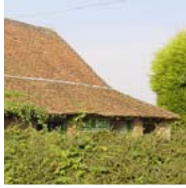
Ashmansworth. Red clay tiles are a traditional roofing material.
