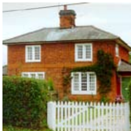
Stratfield Saye. Distinctive casement windows.
