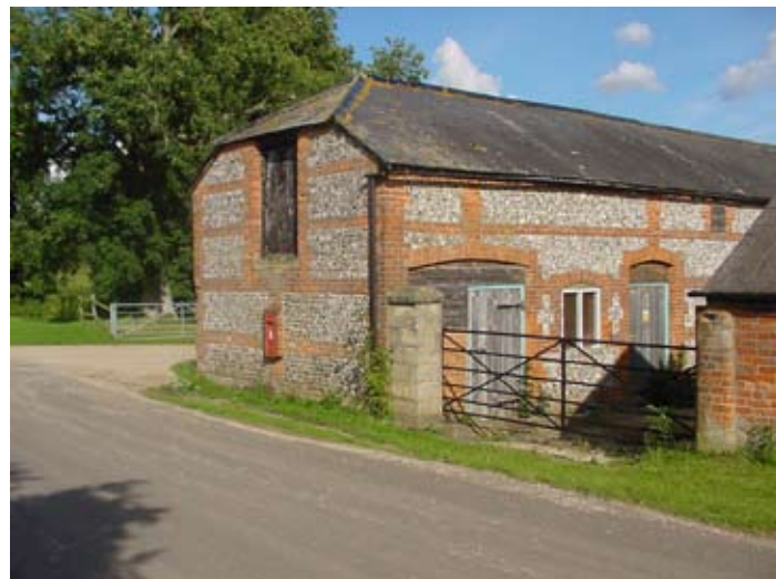
Brick and flint farm building with a half-hipped slate roof, Egbury
