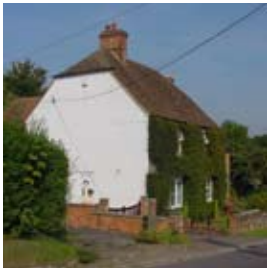
Highclere. Half-hipped roof with red clay tiles.
