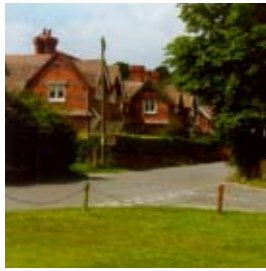
East End. Vertical clay tile hangings.
