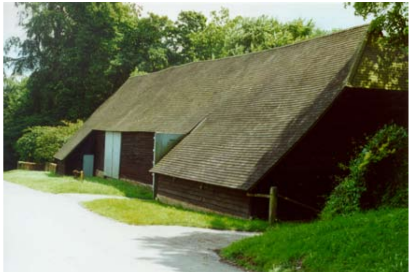
Timber-framed barn with weatherboarding (Tunworth)
