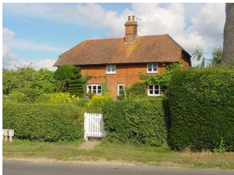
Half-hipped clay tile roof, Old Basing
