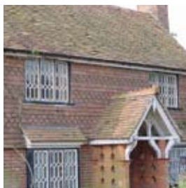
Bramley. Clay tile hanging.
