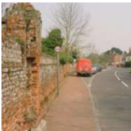
Old Basing. Brick boundary wall and buildings.
