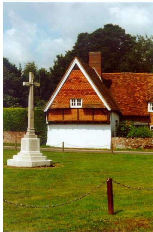
Vertical clay tiles and a red clay tile roof by the village green in East End
