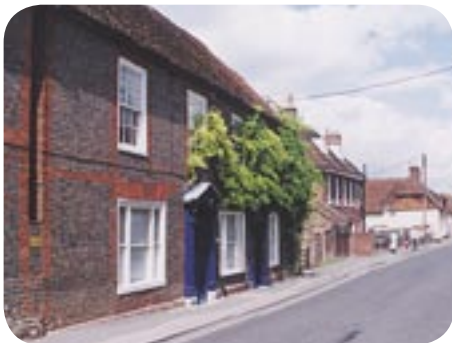
View northwards along Swan Street
