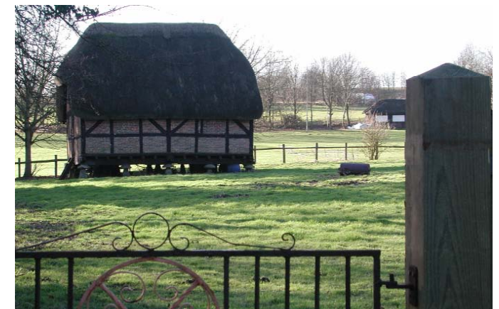
Thatched storage barn sits beside the cricket field off Church Street
