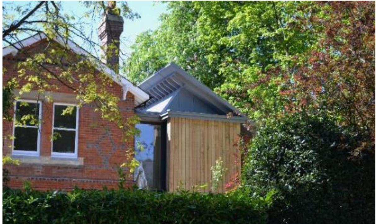
Example of contemporary extension in Winchester which utilises high quality materials and detailing.
