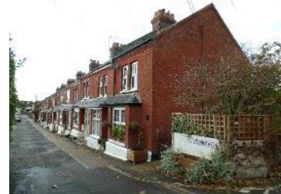
Figure 8: Battens Avenue, Notable Structures
