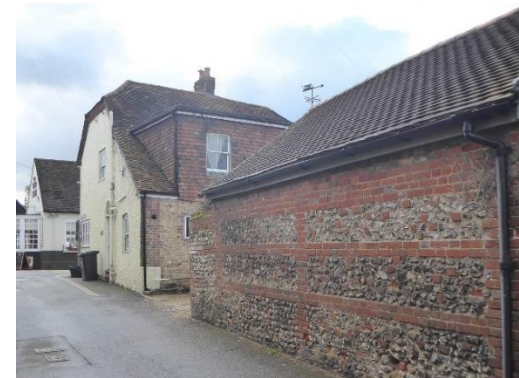
Figure 20. Fox House and outbuilding, High Street, Notable Structures. House is rendered to front and side, flint to rear. Photograph used with kind permission of the copyright owner.
