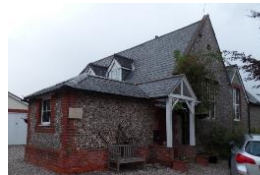
Figure 21. 8 Red Lion Lane, Notable Structure and a landmark (formerly the Infants School). Flint with brick dressings.
