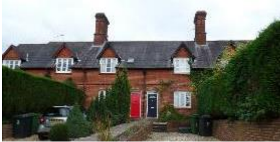
Figure 61. 1-7 Vinns Lane. Notable Structures with large chimneys. 1 ½ storeys in height.
