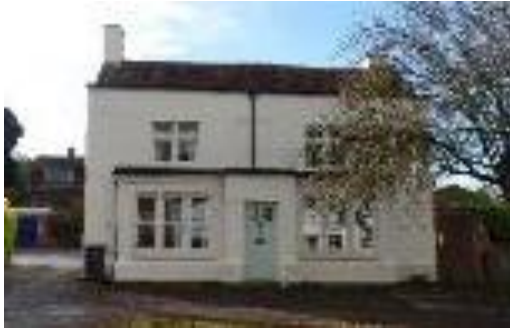
Figure 25. 30 Winchester Street, Notable Structure. Parapet roof.
