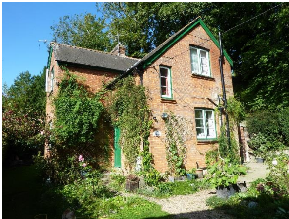
Figure 39. Glebe Cottage, Notable Structure, early C20th, 2 storey house on Glebe Meadow.
