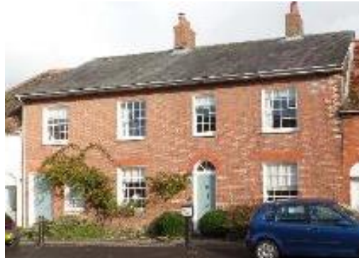
Figure 19. 33 and 35 Winchester Street, Grade II listed, Flemish bond brickwork, with blue brick headers.
