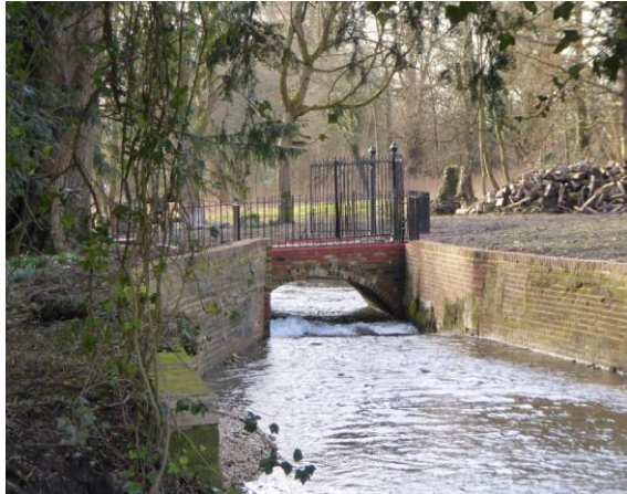
Figure 67. Sluice in grounds of Southington House. Notable Structure.
