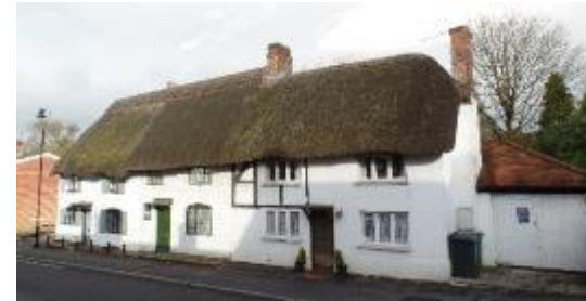
Figure 24. 73, 75 and 77 Winchester Street, Grade II listed landmark. Half-hipped thatched, timber- framed and rendered building. Prominent brick chimneys.
