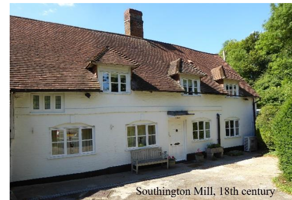
Figure 10: Southington Mill, Grade II listed, landmark, C18th, early C20th. Photograph used with kind permission of the copyright owner.
