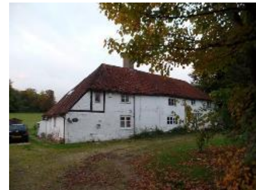
Figure 43. Old Manor, Grade II listed. 17th and early 19th century, timber framed, painted brick. Low outshots. Large chimney.
