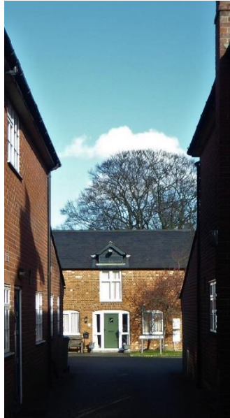
Figure 26. Trimms Court, Notable Structure. To rear of 12 and 20 High Street.
