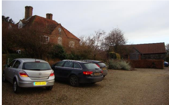
Figure 50. Single storey outbuilding at Polhampton Farmhouse, Grade II* listed.
