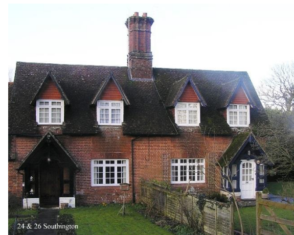
Figure 60. 24 and 26 Southington, former Portals cottage. Notable Structure. Large chimney stack, prominent porches and gabled dormers. Photograph used with kind permission of the copyright owner.
