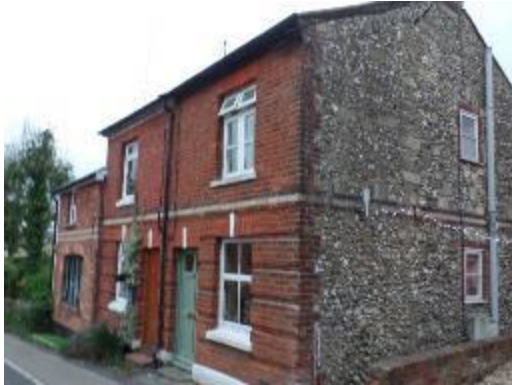
Figure 22. 41 Red Lion Lane, Notable Structure, flint to side elevation.
