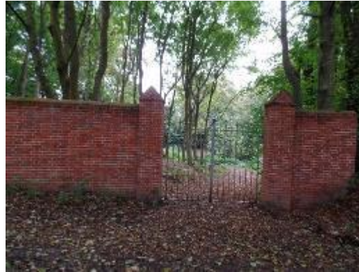
Figure 63. New gates and wall to Southington House from Silk Mill Lane.
