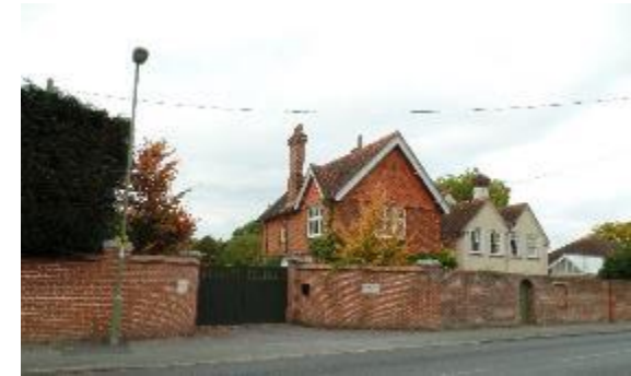
Figure 66. Southington House, London Road. Notable Structure.
