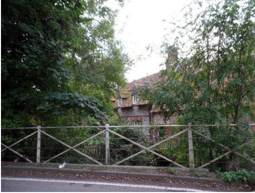
Figure 51. Bridge railings at Quidhampton Mill, Notable Structure.
