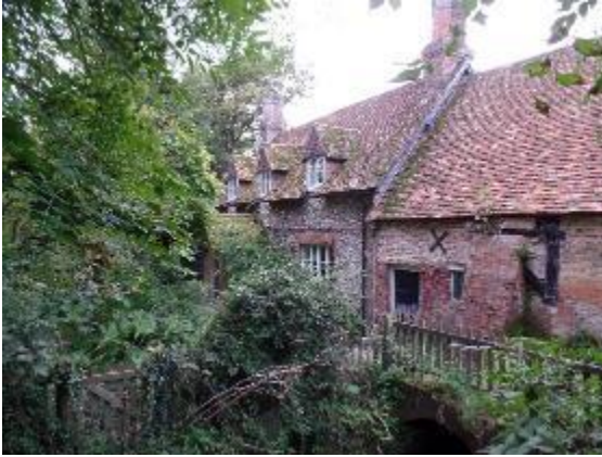
Figure 11: Quidhampton Mill and Millhouse, Grade II listed, landmark, C17th, C18th and mid C19th.
