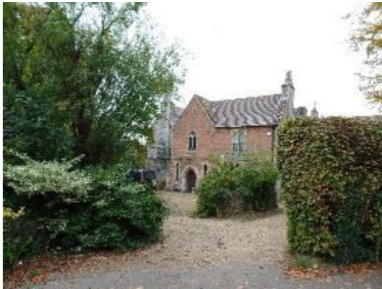
Figure 37. Glebe House, Grade II listed, landmark. On site of earlier rectory, C19th Gothic. Steeply pitched roof, prominent gables, octagonal Tudor chimney stacks, Brick, clay tile, flint rear wing, fine stone dressings.
