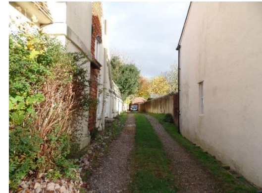
Figure 15. Gap to side of Yield House, 57 Winchester Street, Grade II listed, curtilage listed walls.
