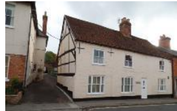
Figure 10. 18 George Street, Landmark building, Grade II, timber frame to side elevation.
