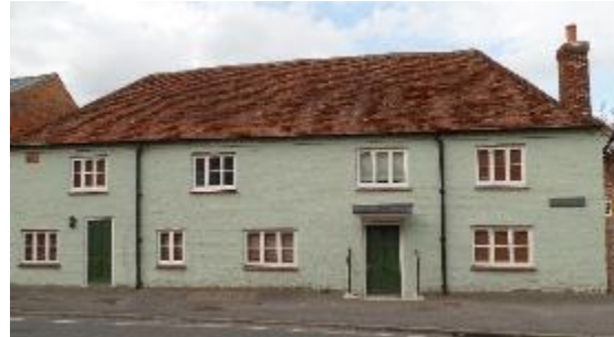
Figure 3. 20 Swan Street, Grade II* listed. Late C14th, C16th, C18th. A timber-framed 2-bay medieval hall, with a 2-bay cross-wing (solar above buttery) at the north side (on right in photo).
