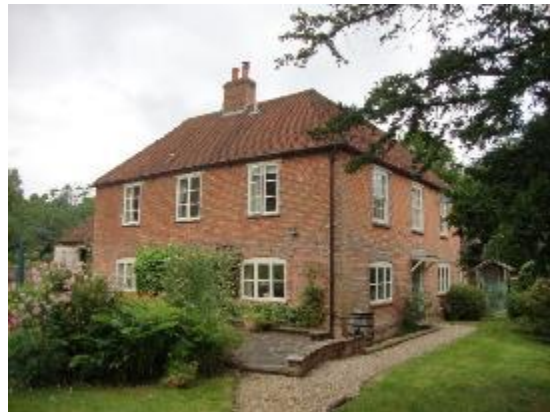
Figure 46. Field Gate Farmhouse
