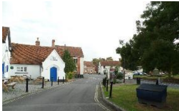
Figure 23. Traditional, black, cast iron posts mark the boundary outside the Crown Public House, Grade II listed. The mature trees in St Mary’s Churchyard are visible to the right of the photo.
