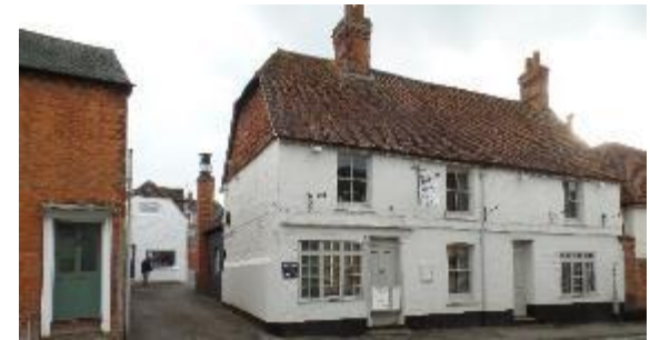
Figure 20. 1 ½ storey outbuilding to rear of 12-10 George, Grade II listed.
