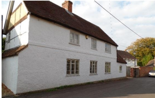
Figure 42. 13 North Street, Grade II listed.
