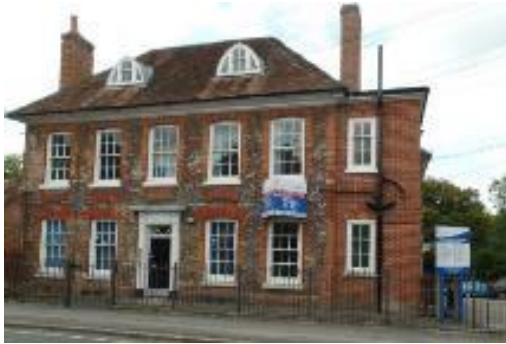
Figure 14. 24 Swan Street, Grade II listed, Queen Anne house, with gothic dormers. Was the Council offices, now let as dance studio and offices. Mild steel railings to road frontage.
