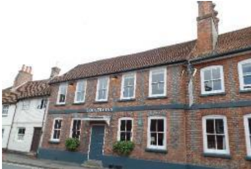
Figure 4. The Swan Hotel, Grade II listed, early C18th, symmetrical Queen Anne design, with prominent chimneys.
