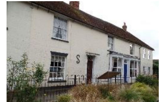
Figure 24. Steel railings in front of 1, 1a and 1b Swan Street, Grade II listed buildings.
