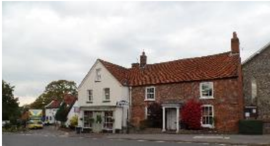
Figure 22. 1 George Street, Grade II listed, prominent gable end facing the road.
