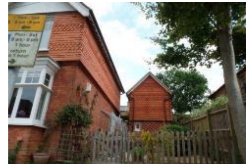
Figure 29. 31 Swan Street, former bank and outbuilding.
