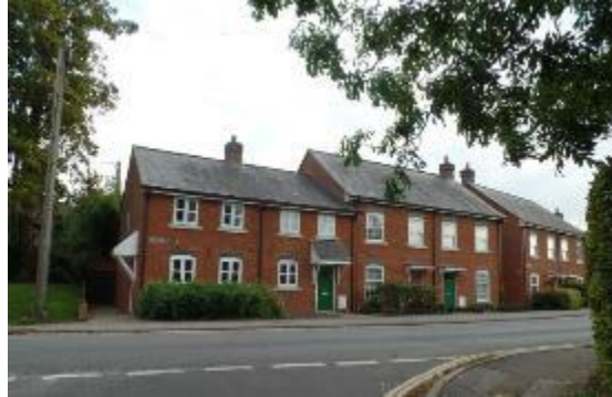
Figure 50. King Alfred Terrace on Ashford Hill Road, B3051.
