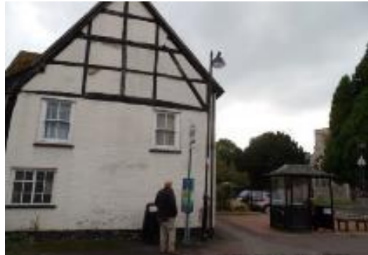
Figure 8. 1 Swan Street, Grade II. C17th and C19th, timber frame partially exposed, painted brick.
