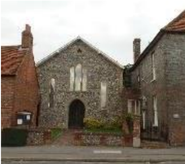
Figure 19. Methodist church, Grade II listed, dated 1809, square knapped flint. Attractive lawn, hedging and wall.
