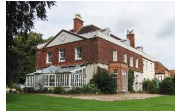
Figure 5. Kingsclere House (with Lake House to rear), Grade II listed: an early C19th 2½ storey large house in extensive grounds.
