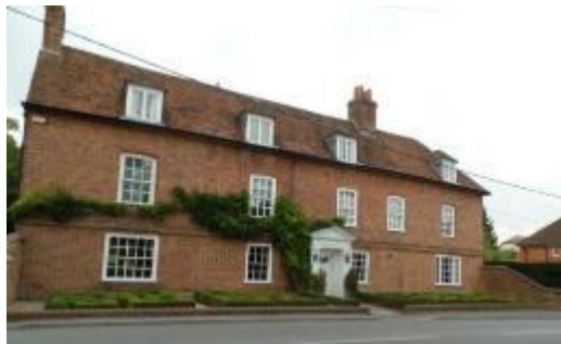
Figure 41. 9 Newbury Road, Grade II listed. 2 ½ storey
