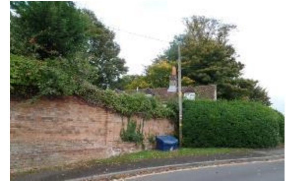
Figure 51. Lodge Cottage roof and the Elm Grove boundary wall on Love Lane.
