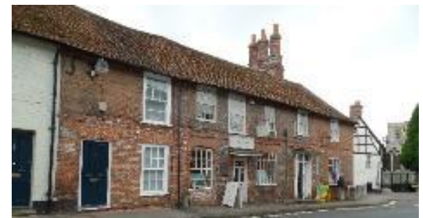
Figure 21. 2 George Street, Grade II listed. Timber-framed building re-fronted in brick. Tudor chimney. Steep roof pitch may indicate a formerly thatched roof.
