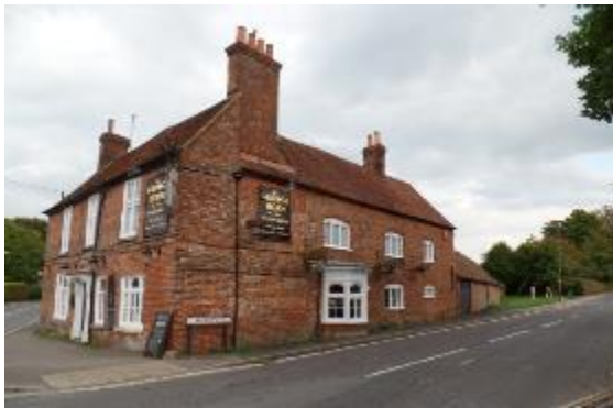
Figure 48. George and Horn Inn, Grade II listed, it has a C17th core. This is a Landmark Building.
