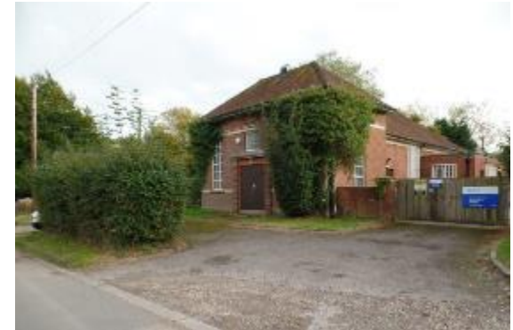
Figure 34. 1930s Water works, a BOLI, on Bear Hill
