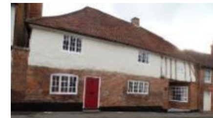
Figure 18. 8 George Street, Grade II listed, rendered with timber frame exposed in part.
