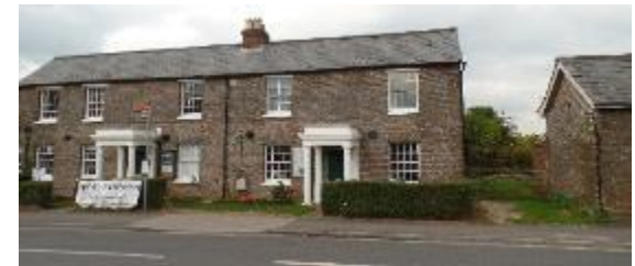
Figure 9. 35 and 37 George Street, Grade II listed. Built 1832. Ornamental blue bricks in header bond with Tuscan porches. 39 and 41 George Street, (to right), also blue brick.
