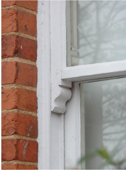
Figure B3a: Detail of a single-glazed timber sliding sash window
