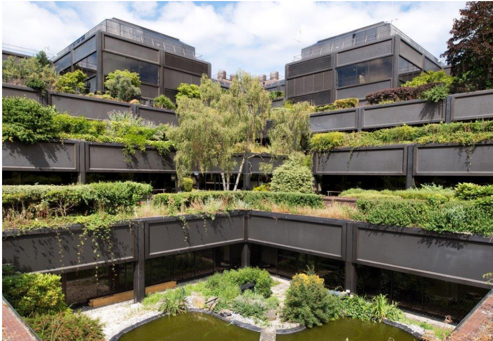
Figure 8: Roof Gardens, Mountbatten House, part of a landscape on the Register of Parks and Gardens
