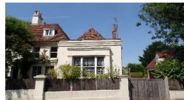
Figure 53. Benwells, Church Street (Grade II listed) is 2 ½ storeys tall with a single storey wing (with parapet).
