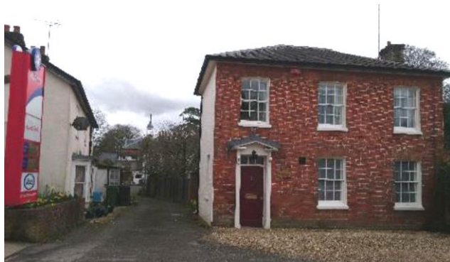
Figure 31. 17 Church Street, Grade II listed. Glimpsed view of Silk Mill Tower to the left.
