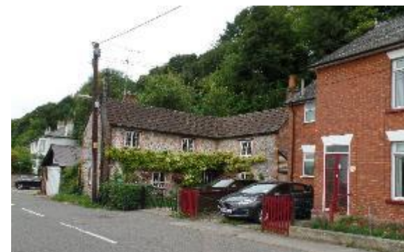
Figure 88. 69 London Road, Notable Structure with two telegraph poles and two street lights.
