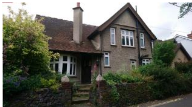
Figure 42. 1 Oakland Road, Notable Structure.
