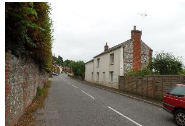
Figure 87. 96 London Road, Notable Structure. 3 storeys on to Pound Meadow.
