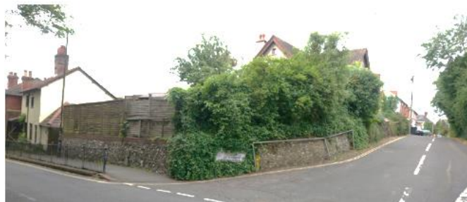
Figure 43. Wall at 1 Oakland Road, Notable Structure.
