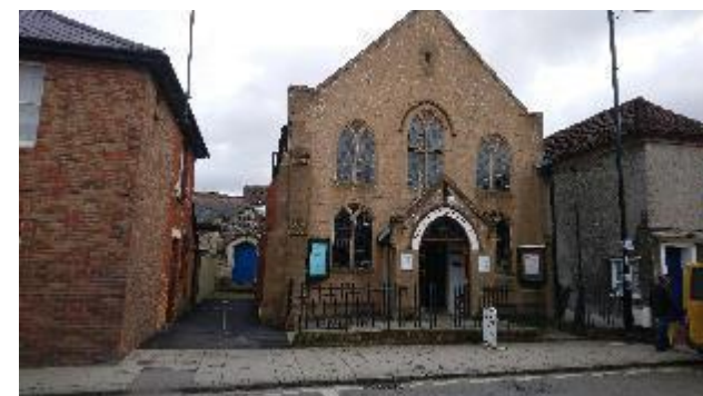
Figure 14. Methodist Church, Winchester Street. Building of Local Interest.
