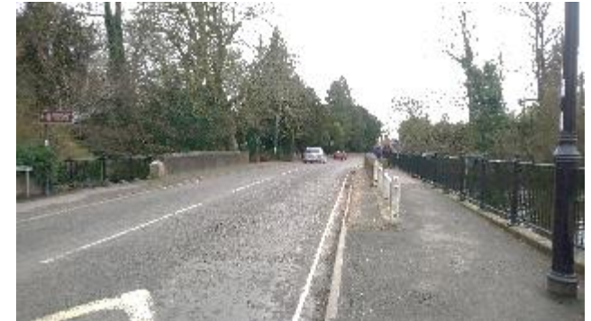
Figure 78. Roadside walls and metal railings on Great Town Bridge, Winchester Street. Notable Structures.
