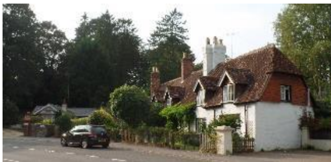
Figure 58. The Hermitage and The Cottage on Church Street, Grade II listed. Mount Lodge to the left is a Notable Structure.
