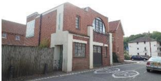
Figure 26. Parapet at Gryphon House, Bell Street, Notable Structure.
