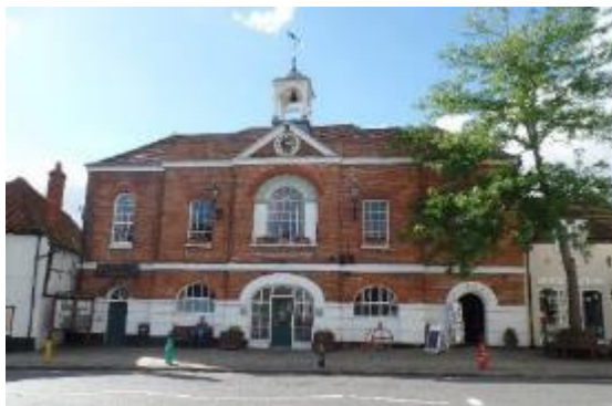
Figure 5. The Town Hall, Grade II*. Dates from the late 18th century.
