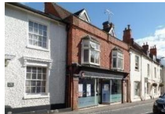
Figure 24. Parapet at 2 Newbury Street, Notable Structure.
