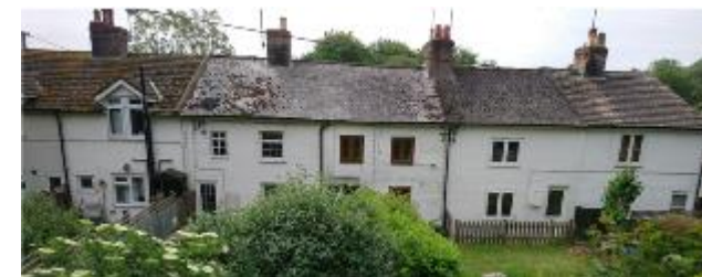
Figure 89. 1-6 Pound Meadow, Notable Structure. View from London Road.
