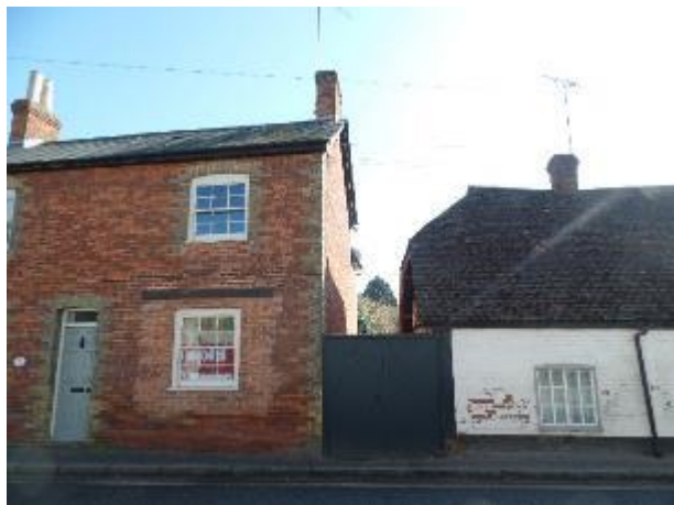
Figure 16. Gap between 32 London Street (Grade II listed) and 36 London Street, Notable Structure.
