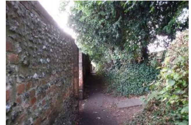
Figure 93. Brick and flint wall to the east and north of 20 to 23 Chatter Lane, Notable Structure.
