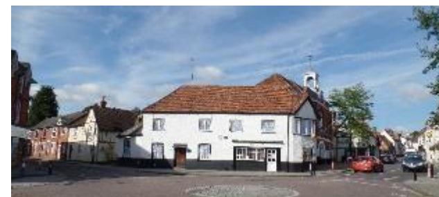
Figure 20. The Bee Hive at 2 Bell Street, now white rendered is timber framed. 15th-century Grade II listed building.
