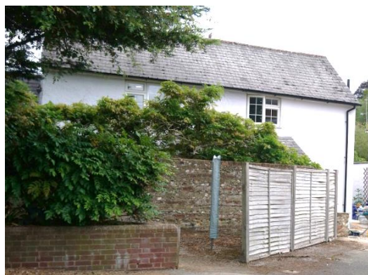
Figure 45. Brick and flint boundary wall south of Yeomans Cottage, Lord Denning Court off Newbury Street. Notable Structure.
