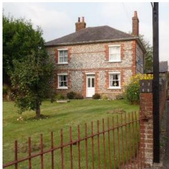
Figure 22. 38 Bell Street. Flint former Farmhouse. Notable Structure.
