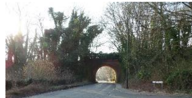
Figure 74. The railway bridge over Church Street, Notable Structure.
