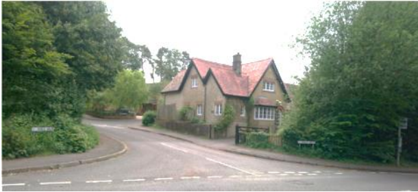
Figure 47. The Lodge, Kings Walk, view from Newbury Road. Notable Structure.
