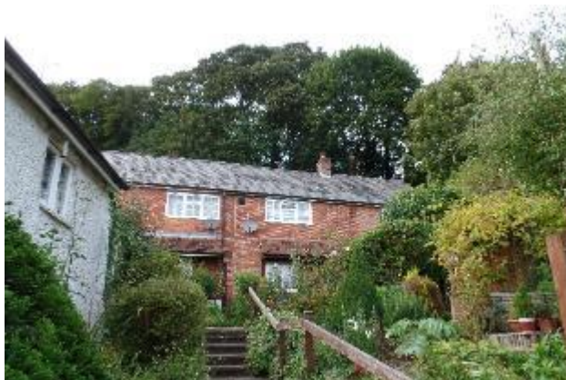
Figure 83. 1 and 2 The Lynch, Notable Structures, looking north toward the Important Open Space (IOS) trees at Bere Hill.
