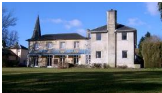
Figure 54. The Lawn, Grade II listed. Late 19th, early 20th century. Plain, symmetrical Grecian façade to east, 20th century extension.
