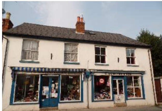
Figure 17. Traditional shopfront at 12 Bell Street, Notable Structure.
