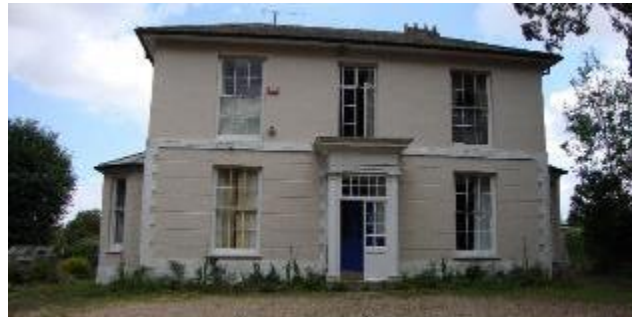
Figure 67. Red Leaf House, Winchester Street. Grade II listed.
