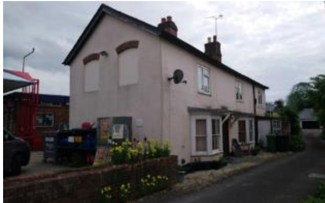
Figure 38. 13 Church Street. Notable Structure.
