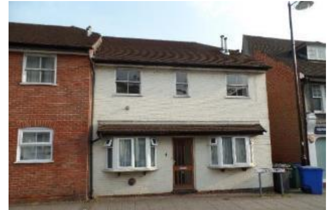
Figure 32. 3 and 4 Waterloo Court, London Street.
