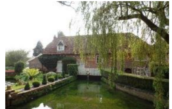
Figure 9. Fulling Mill, Grade II listed.
