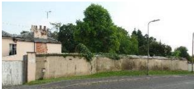
Figure 60. Cob boundary wall, curtilage-listed at The Mount, Wells Lane. Important Open Space (IOS) trees in the background.
