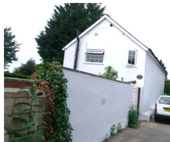
Figure 44. Yeomans Cottage. View from Boundary Close. Notable Structure.
