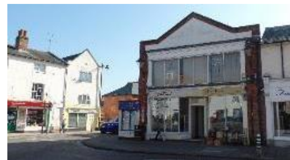
Figure 25. Gabled parapet at 1 Church Street, Notable Structure.
