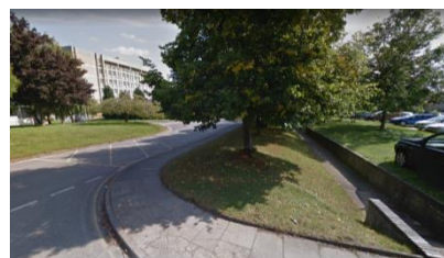
Figure 24: Hospital duct run along verge of Dinwoodie Dr
