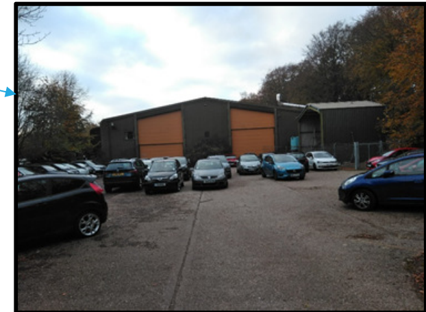
Figure 2.1.3 ECB – ex-laundry site
