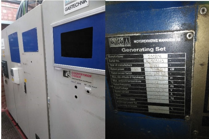
Figure 17 The acoustic casing for the CHP (left), and the CHP plate (right)
