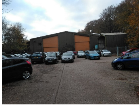
Figure 11 The unused laundry building, with an old gas connection evident on the right of the photo
