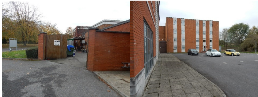
Figure 25 the entrance to the area next to the car park where the plantroom can be accessed (left), car park that would need to be crossed (right)
