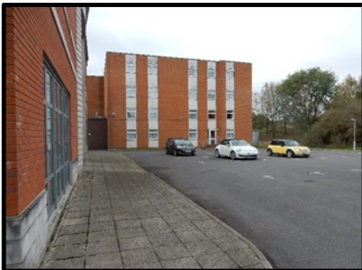
Figure 1.7.1 Hotel building fabric and carpark that will need to be crossed
