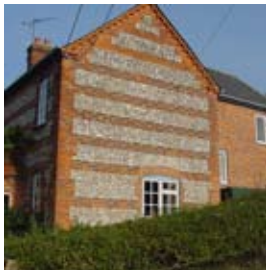
Binley. Bands of brick and flint, with a dentil course of bricks below the gabled roof.
