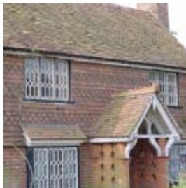
Bramley. Clay tile hanging.
