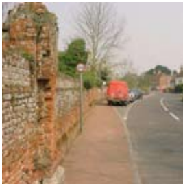
Old Basing. Brick boundary wall and buildings.
