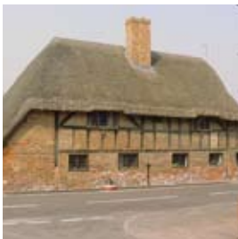
Old Basing. Timber frame and thatch.
