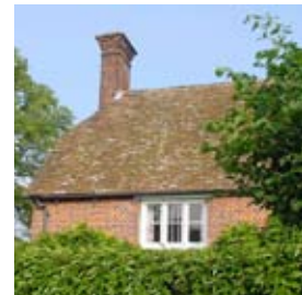
Stoke. Traditional casement window and chimney detail.
