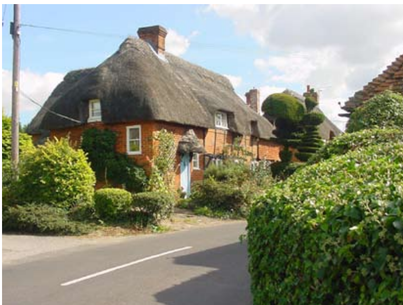
Timber framed and thatched house in Old Basing
