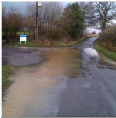
Picture 2 Shows run-off complete with sediment flowing down Minchens Lane
