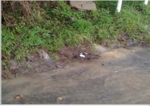
Picture 1 Shows water running off the fields at the start of the "Electricity Road" after heavy rain. The water is not fed to the culvert or ditch but flows down the road laden with sediment.
