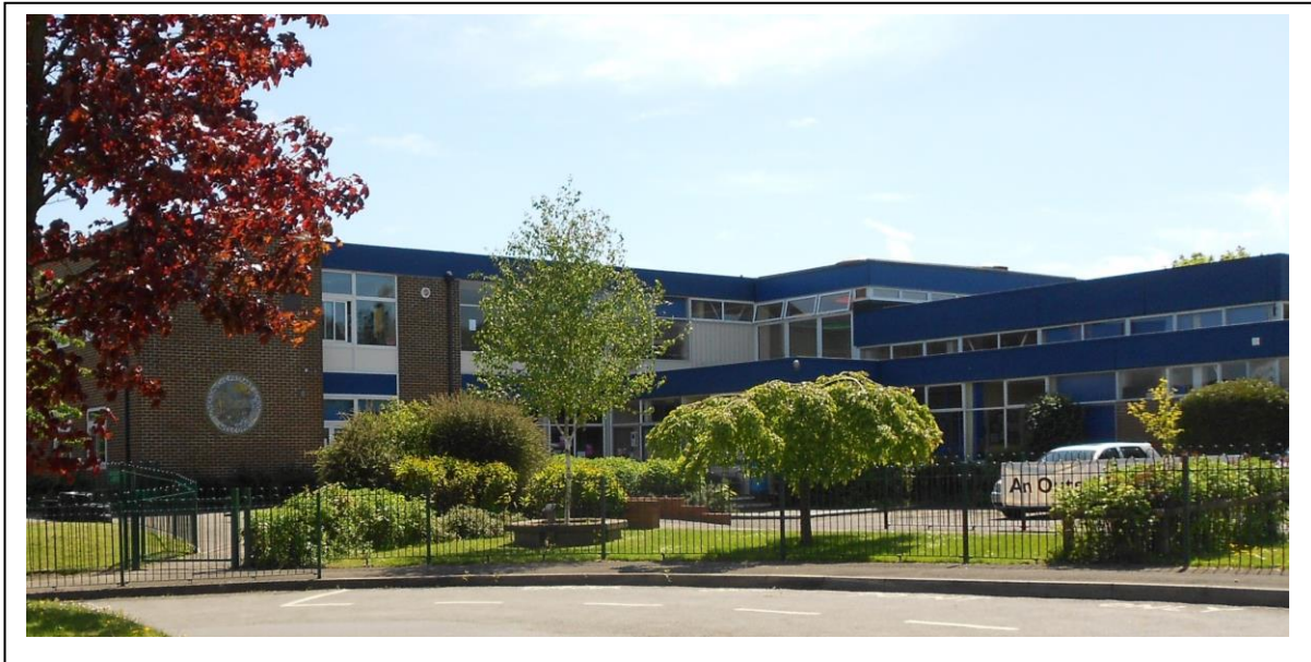
Overton Primary School at Court Drove
