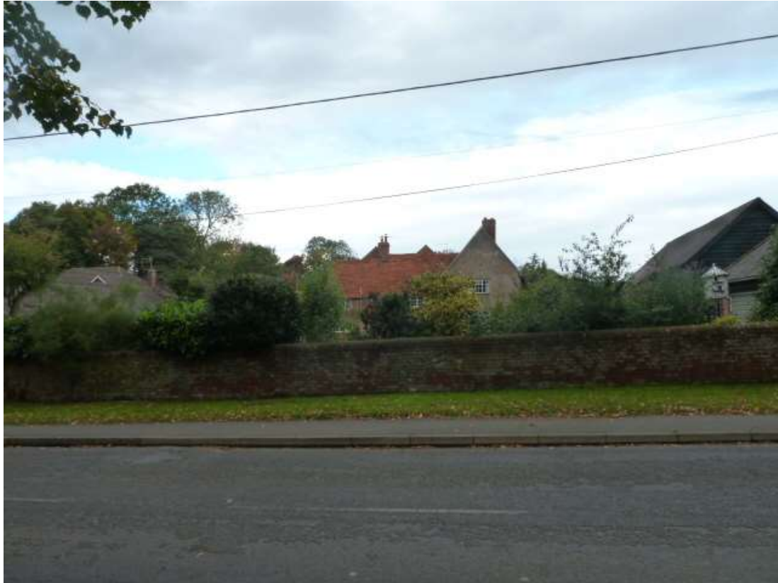
5. Cranes Farmhouse (Listed) from the Southside of Cranes Rd.
