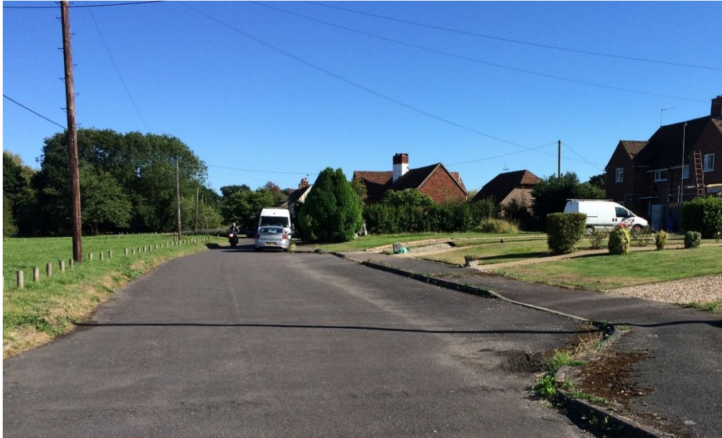
Figure 4-6 Parking layby in The Plantation
