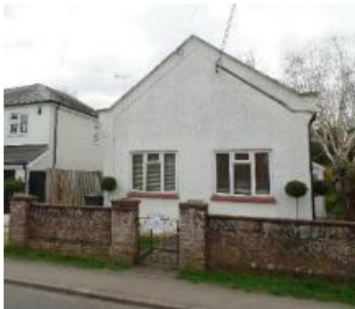
Figure 64. Former Congregational Chapel, 15a Pyotts Hill, Notable Structure.
