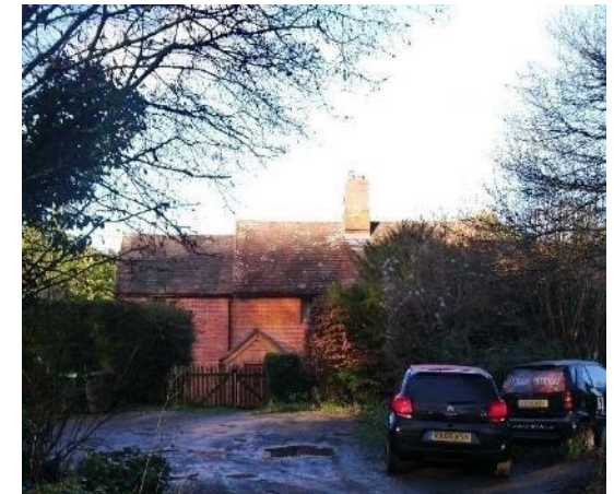
Figure 70. 1 & 2 Swing Bridge Cottages, Notable Structures.
