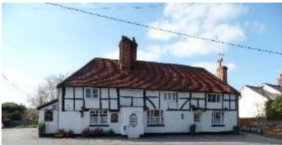
Figure 24. Bolton Arms Public House dates from the 16th, 17th and 19th centuries. Grade II listed.
