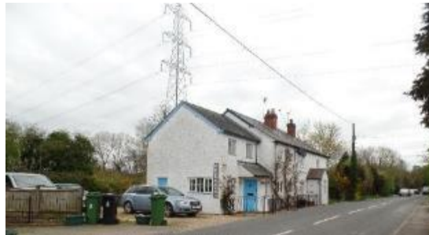
Figure 65. 2 & 4 Pyotts Hill, Notable Structures.
