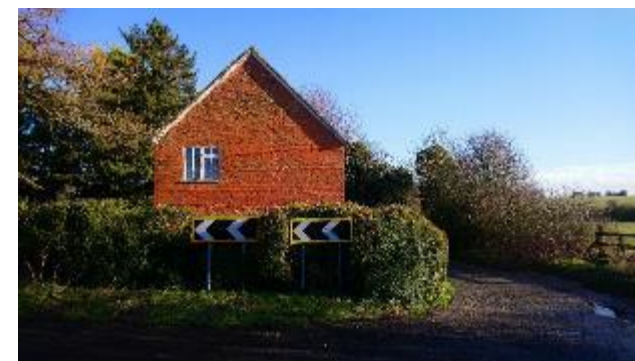
Figure 49: Redbridge Cottage. Notable Structure.
