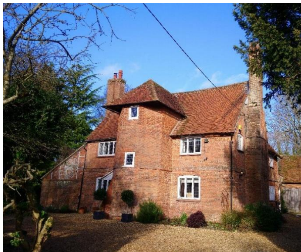
Figure 29. Parkers Farmhouse. Octagonal stair turret. Grade II listed.
