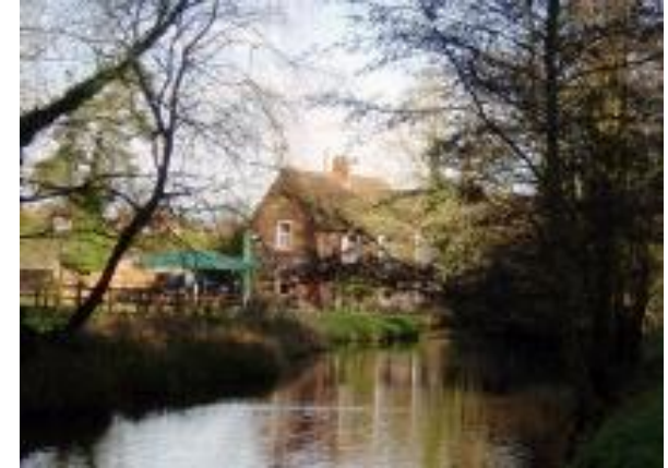
Figure 14. Barton Mill Public House and restaurant (Grade II listed). Late 17th, early 19th centuries. View from Public Footpath No.20 to the southwest.
