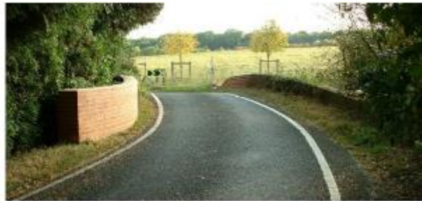
Figure 17: Redbridge Lane Bridge over the canal (was formerly known as Slaughter Lane Bridge). Notable Structure.
