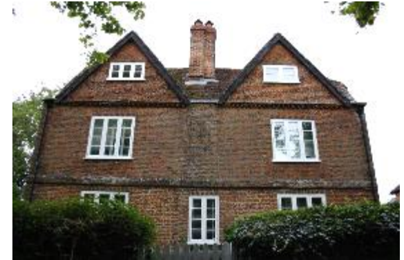
Figure 12: Church Lane House, Grade II listed, formerly The Workhouse, erected in 1836). Walling is in 'Tudor' brickwork of mixed bond.
