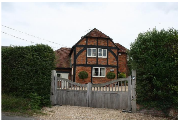
Figure 37. 2 Milkingpen Lane. Grade II listed.
