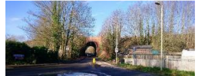
Figure 56. Swing Swang Lane railway bridge (Notable Structure).
