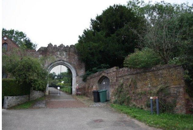
Figure 11: 16th century Garrison Gate the only surviving gate to Basing House, with late-19th century rusticated battlements. Grade II listed.
