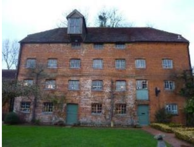
Figure 13. Four storey Lower Mill, Grade II listed. Late 18th, early 19th Century. The tile roof is ½ hipped.
