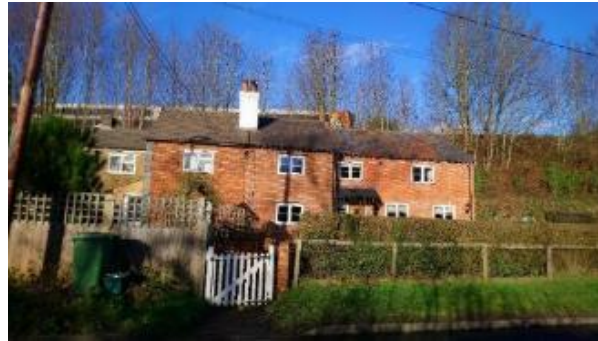
Figure 50. 1 and 2 Railway Cottages, Swing Swang Lane. Notable Structures.
