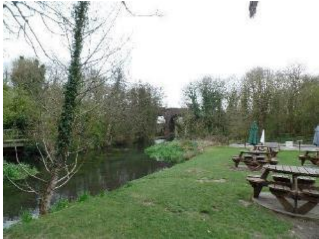
Figure 55. Important Open Space at Bartons Mill, view to railway arches over the River Loddon (Notable Structure).
