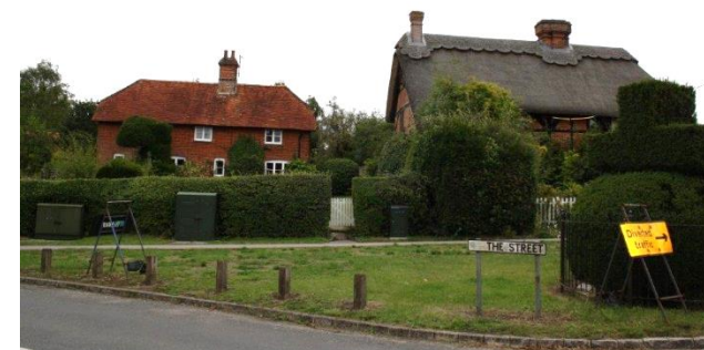
Figure 32: Northern part of the OATS outside 5 Milkingpen Lane (Landmark) 16th century, 2 ½ storey height gable end. 3 Milkingpen Lane, to the left. Both Grade II listed.
