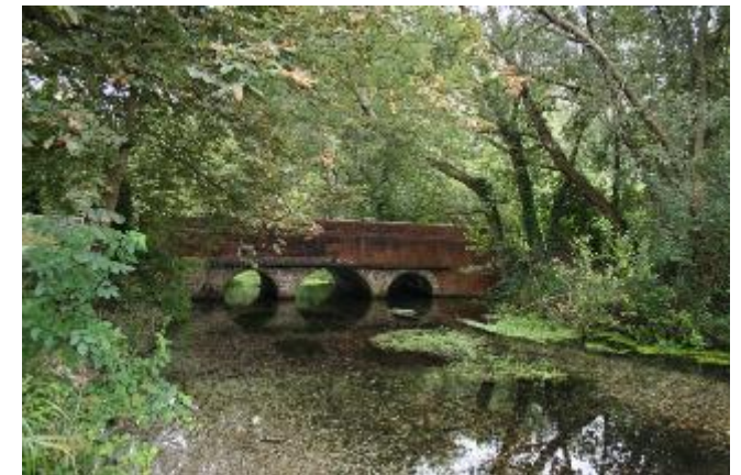
Figure 18: Basing Road bridge over the River Loddon. Notable Structure.
