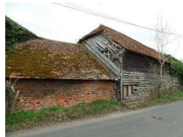
Figure 54. Barn at Lower Mill, view from Newnham Lane. Curtilage listed.
