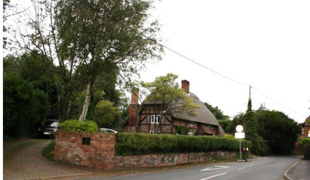
Figure 45: 4 Crown Lane. Grade II listed.
