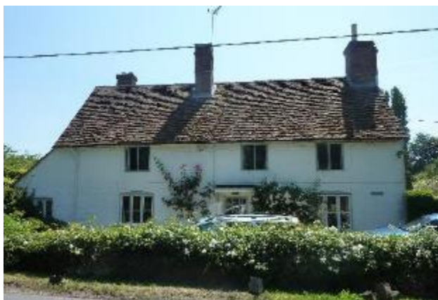
Figure 52. Yeomans, Newnham Lane. Grade II listed, Landmark. Painted brickwork.
