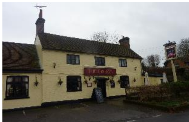
Figure 44: The Crown Inn, The Street. Grade II listed.
