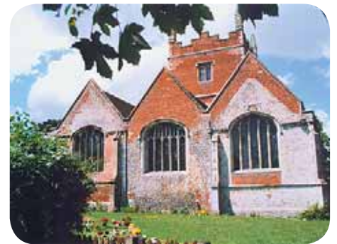
East elevation of St Mary's Church
