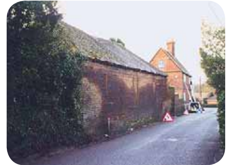
Wall of outbuilding, 2 Crown Lane
