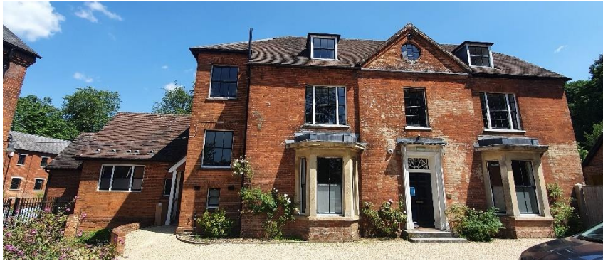
Figure 36. Laverstoke Millhouse. Grade II listed.
