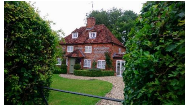
Figure 13. Batts Cottage. Grade II listed.
