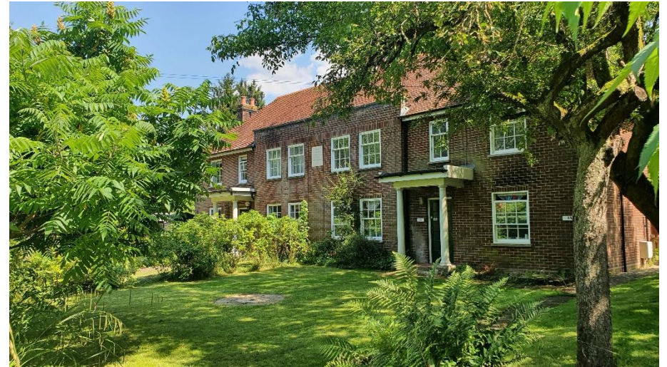
Figure 41: 3&4 Memorial Cottages has a partial parapet.
