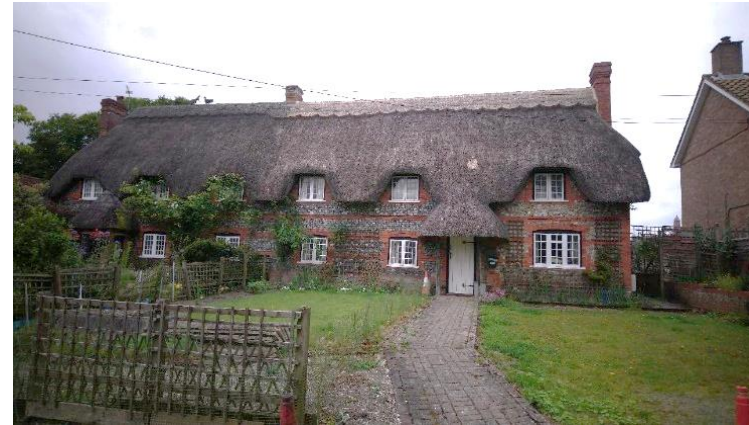
Figure 23. 12 and 14 Priory Lane. Notable Structures.
