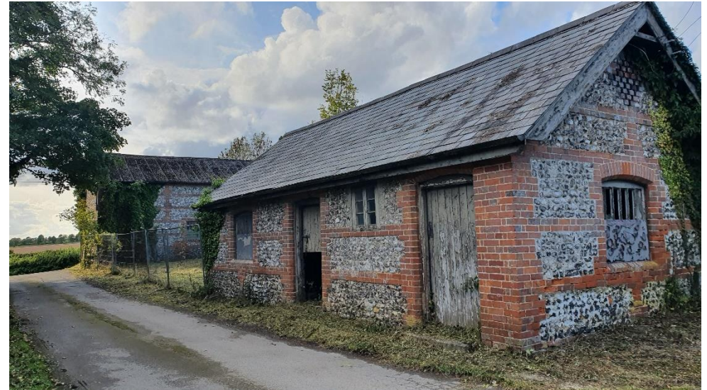
Figure 48. Home Farm outbuildings.
