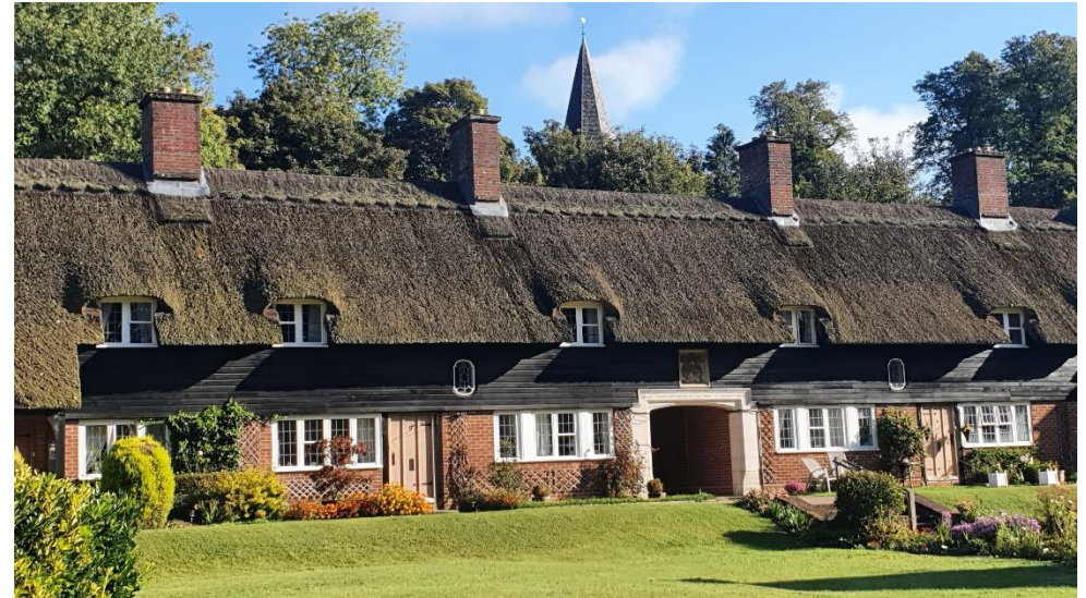
Figure 28. Manor Cottages and St Mary's Church spire (Grade II listed).
