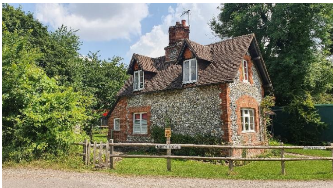
Figure 50. North Lodge. Notable Structure.
