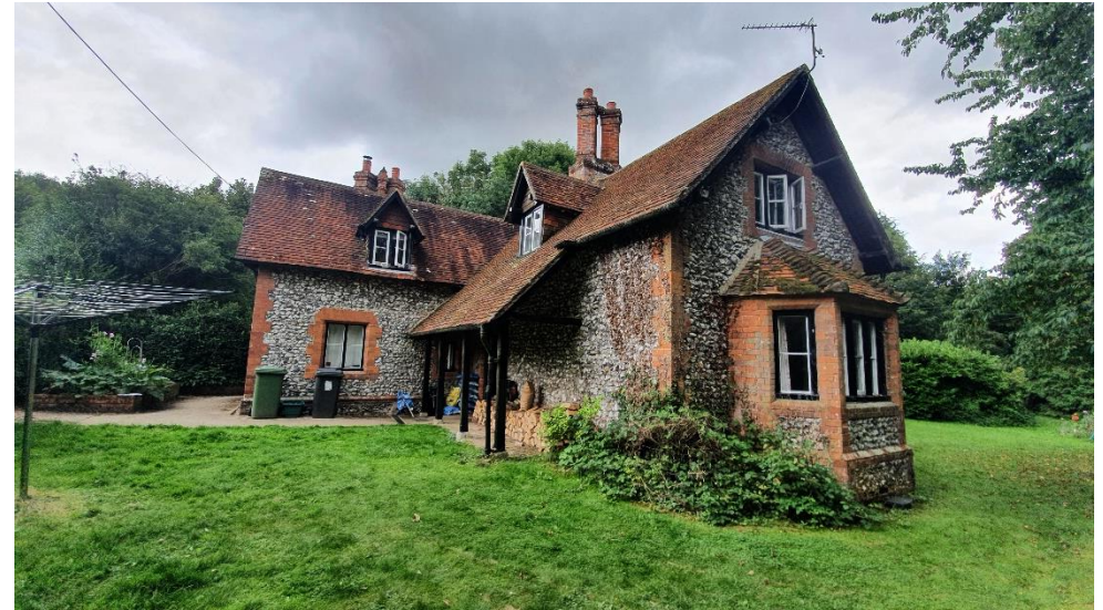
Figure 54. Home Farmhouse. Notable Structure.
