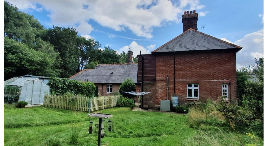
Figure 51. 46 Home Farm Lane. Notable Structure.
