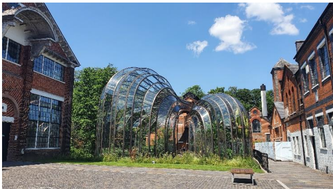
Figure 38. Glass House at Bombay Sapphire Distillery. Former Wheel House and Glazing House on the right are Grade II listed.
