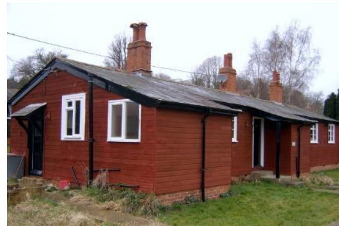
Figure 9. 1 The Bungalows, Laverstoke Lane. Notable Structure.
