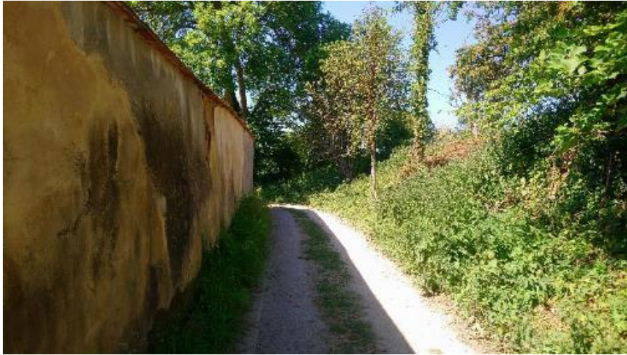
Figure 19. Cob wall at Bere Mill. Curtilage Listed.
