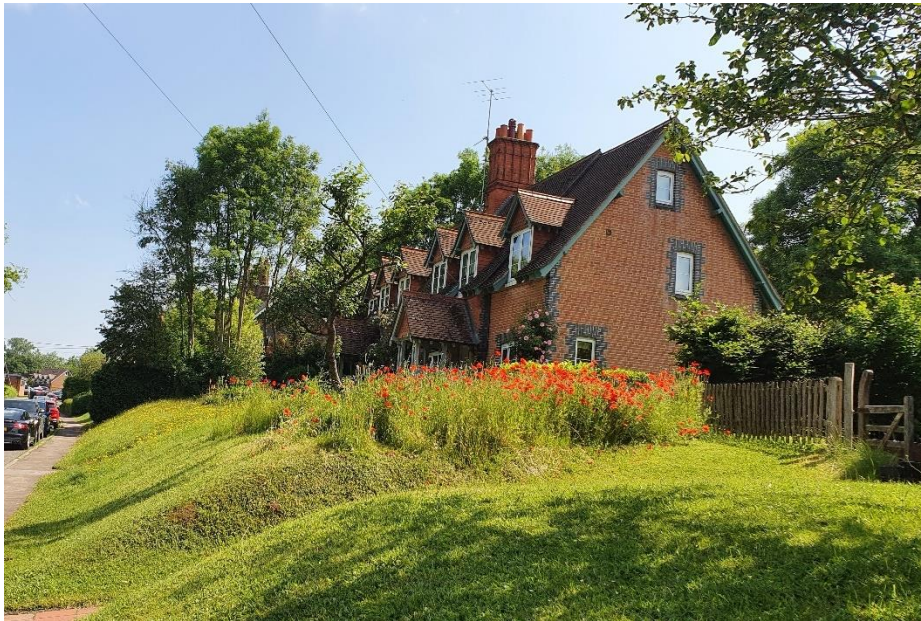
Figure 8. 29 and 30 Laverstoke Lane. Notable Structures.
