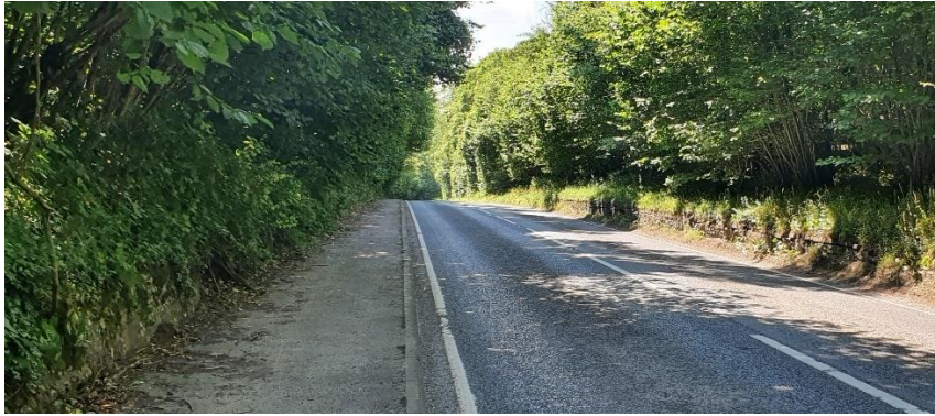
Figure 17. Brick and flint revetment to Rotten Hill, view west. Notable Structure.
