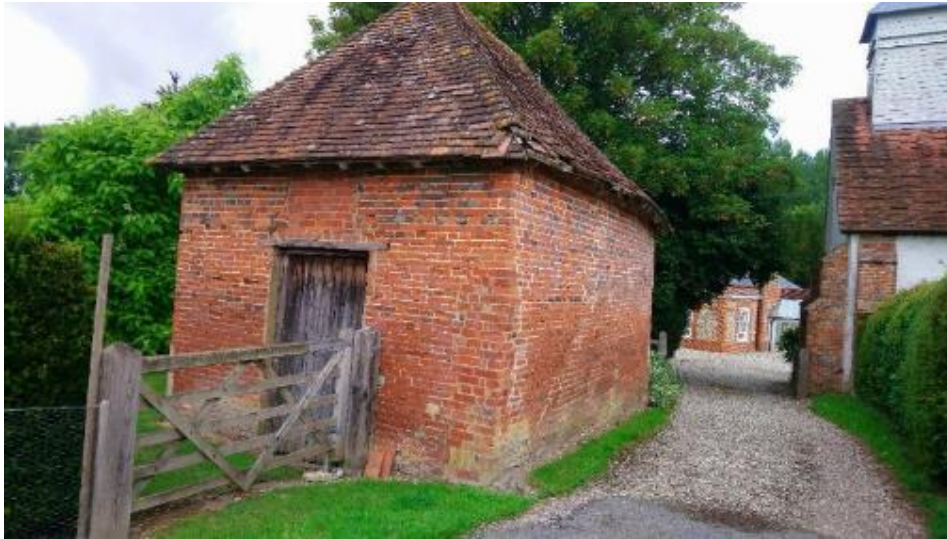
Figure 29. Single storey outbuilding at Manor Farm. Notable Structure.
