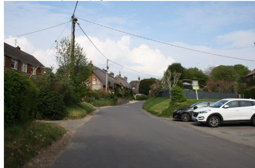
Figure 30: Yew Tree Lane, view east to Yew Tree Cottages. Notable Structures.
