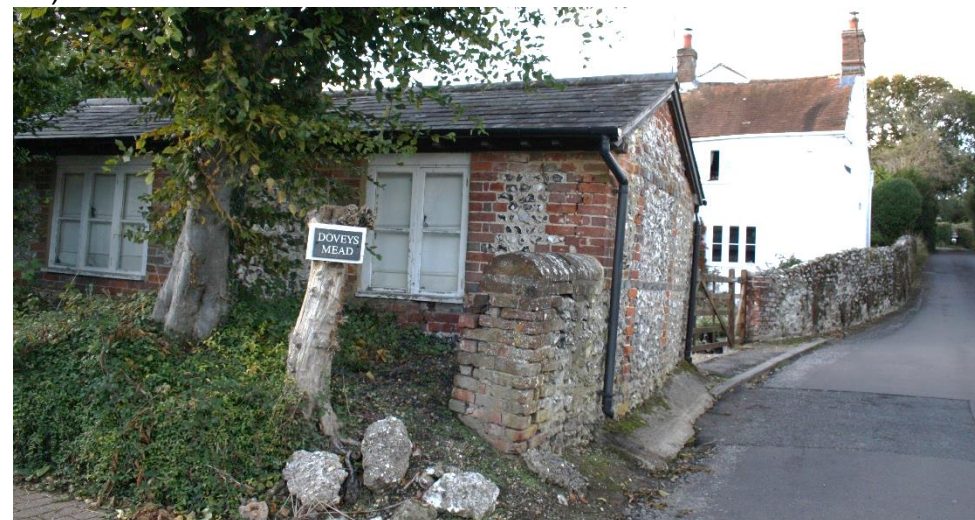
Figure 12. Single storey outbuilding at Holly Cottage, Chapel Street. Notable Structures.
