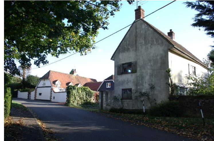
Figure 25: Maiden Thorne Cottage and Towns End Cottage, Up Street. Notable Structures.
