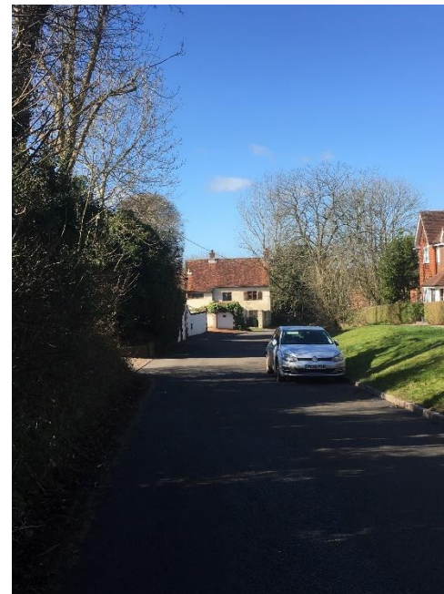
Figure 26: Towns End Cottage, Up Street. Notable Structure.
