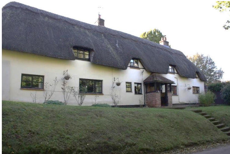
Figure 40: Kyte Abbey, Popham Lane. Notable Structure.
