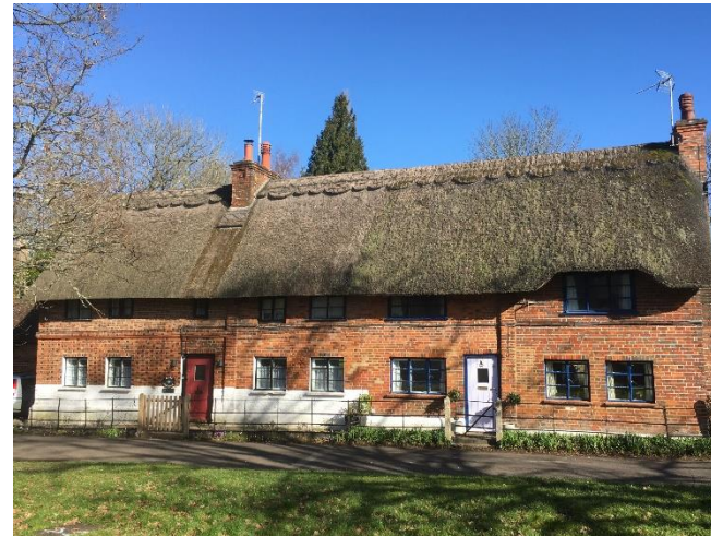
Figure 17. Blake Cottage, Grade II listed.
