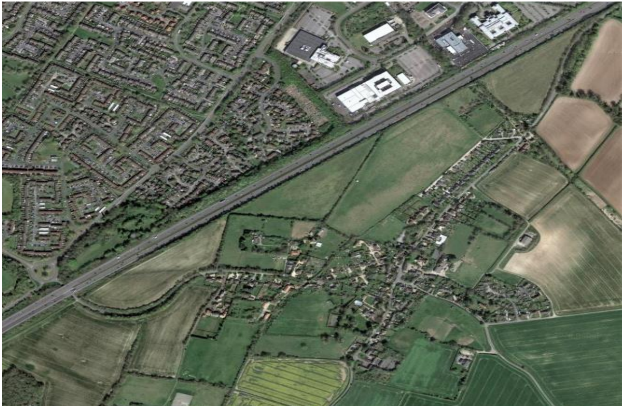
Fig 1: Aerial view of the proposed Local Gap area showing the distinction between Cliddesden parish to the south and Basingstoke town to the north. ref: Google Maps
