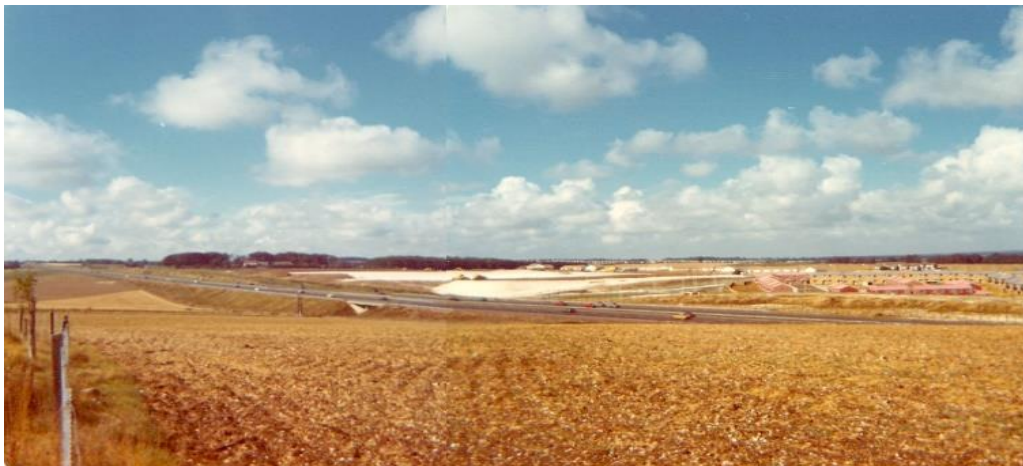
The M3 motorway (1972) under construction
