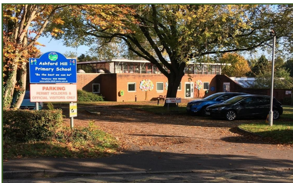
Figure 17 Ashford Hill Primary School
