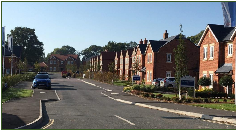
Figure 31 Oakfield Lane, Ashford Hill
