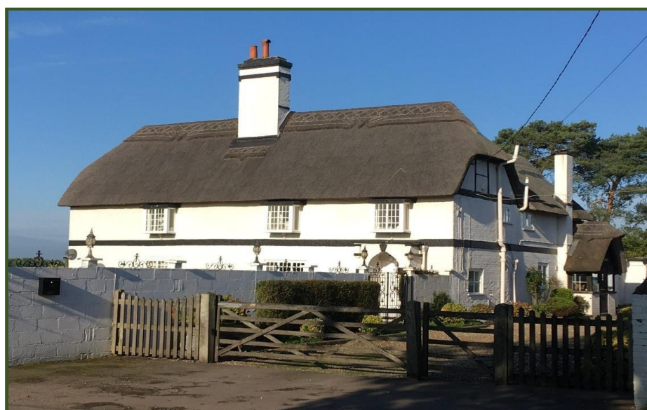
Figure 14 Ashford Hill Farmhouse (Listed grade 2)
