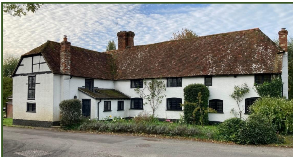
Figure 13 The White House, Galley Lane (Listed grade 2)
