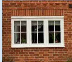
Window muntins and vertical brick details
