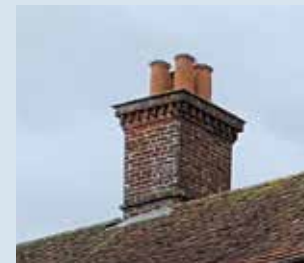
Masonry chimney stack
