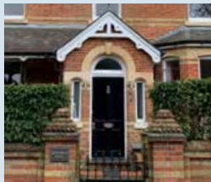
Decorative features on the roof eaves
