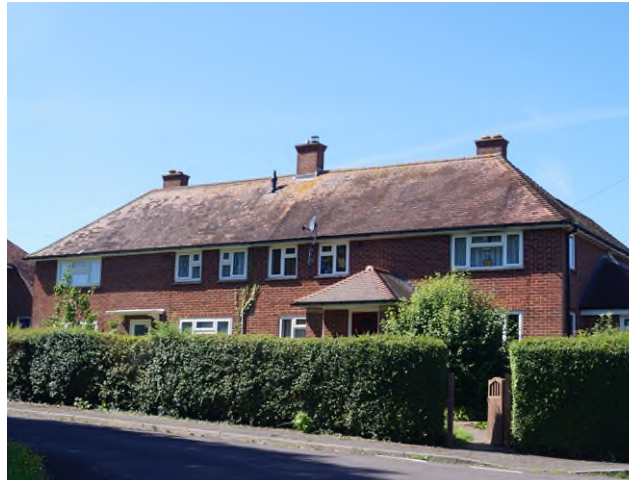
Figure 30: Semi-detached house which is typical to this CA with red brick and a tiled, hipped roof.
