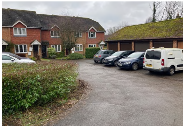
Figure 47: Terraced houses with courtyard parking, Cranesfield, which is somewhat out of character with the rest of the public realm in the village.
