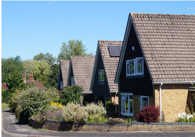
Figure 38: Chalet bungalow typology in Tyfield with steeply pitched roofs.
