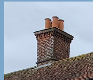
Masonry chimney stack
