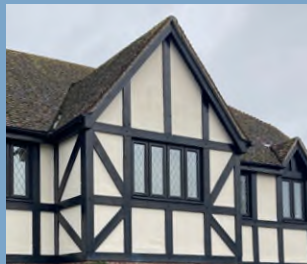
Exposed timber framework
