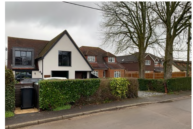
Figure 37: Variable rooflines including hipped and gabled, created by a range of house types and ages, which adds interest and character and is typical of the CA and the Parish as a whole.
