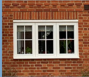
Window muntins and vertical brick details
