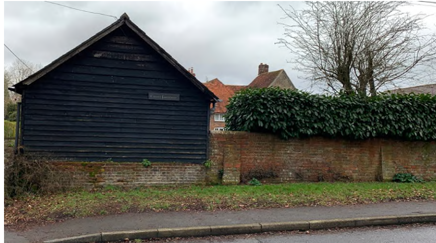
Figure 19: Use of black timber weatherboarding and red brick wall on Cranes Road, which resonates with the prevailing material and colour palette in the CA.
