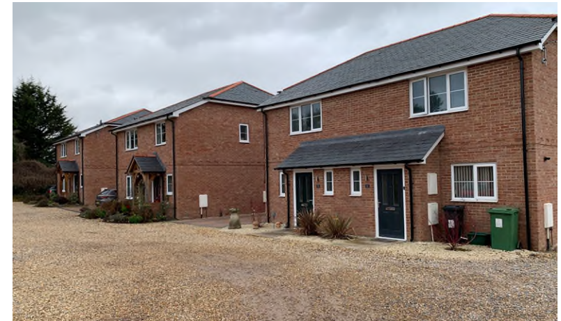
Figure 21: New built semi-detached houses on Aubery Place, which simple casement windows, porch features and material palette are in keeping with the historic character of the CA.
