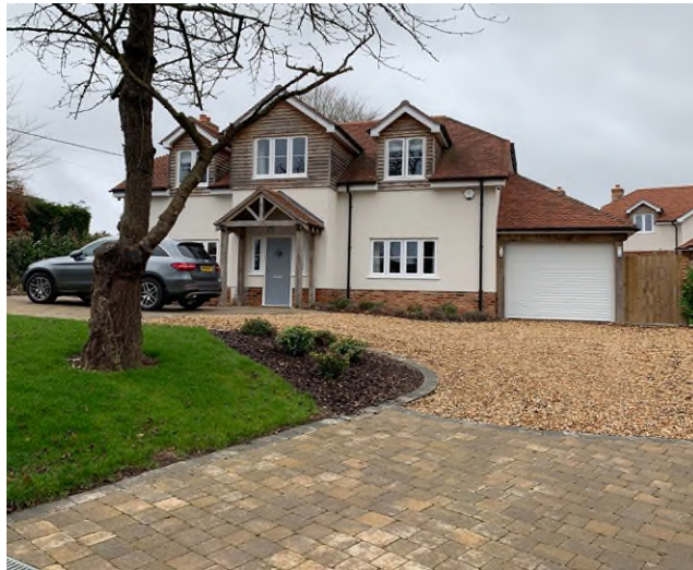
Figure 32: A recently constructed detached house with timber weatherboarding and rendered facade, as well as other features such as the porch and gabled dormers, which reflect the historic character of the village.
