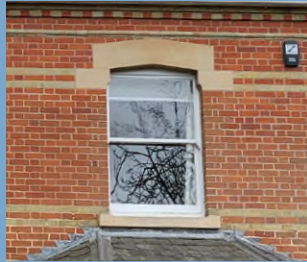
Sash window and fenestration detail
