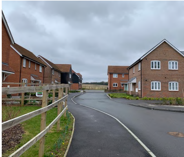
Figure 43: Detached houses, Sireburn Close with clay tile, red brick and timber weatherboarding, in keeping with the historic character of the CA and the village. However due to the small gaps between buildings, short set back distances and use of hard boundary treatments the development has a urban feel which does not fully reflect the rural, village character of Sherborne St John.
