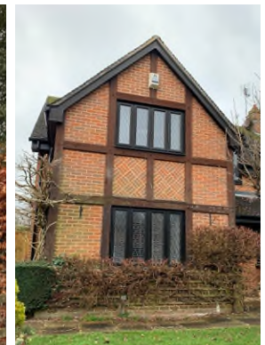
Figure 107: Red brick front, black exposed timber frame
