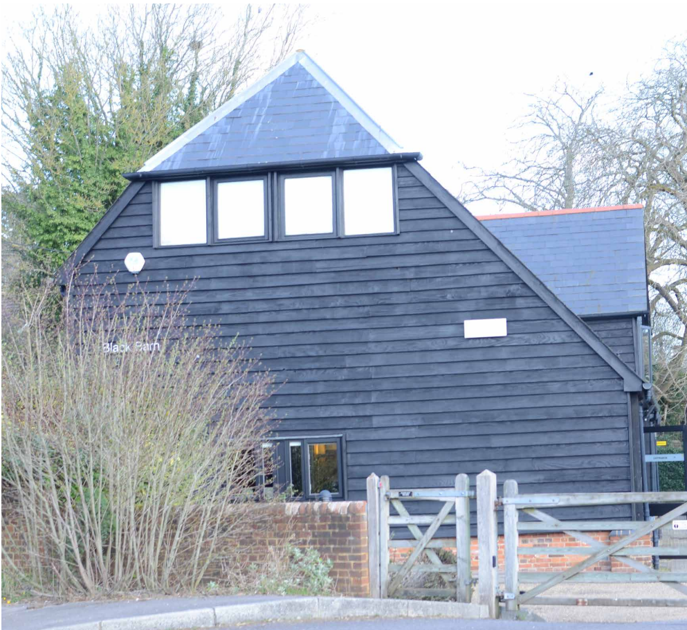
The Black Barn, a converted black weatherboard barn in the Village Core, combines traditional materials with modern detailing to create a distinctive building in keeping with local character
