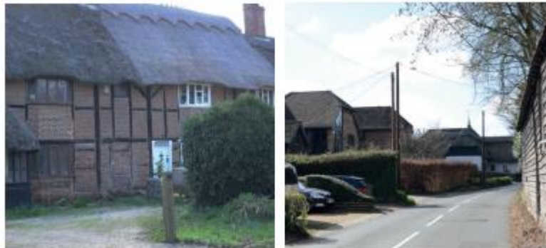
Farleigh Road thatch and barn
