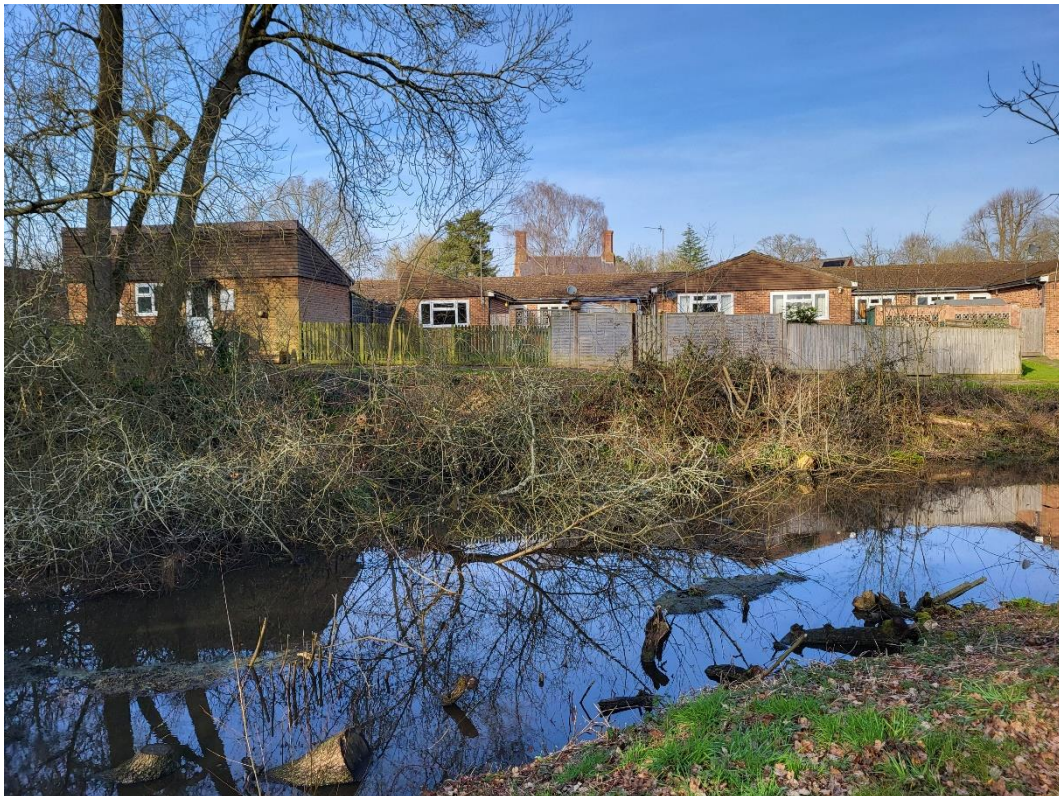
Plate 14: The roof and chimneys of Culham's Farmhouse seen in views across Flex Ditch from Little London Road
