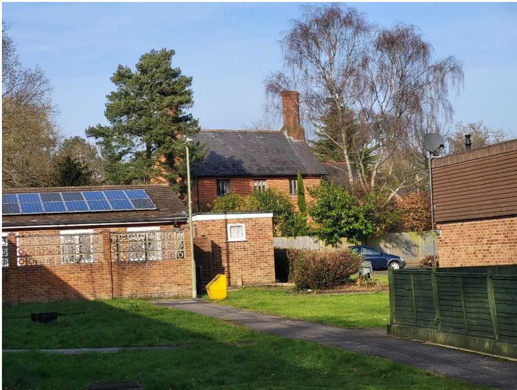
Plate 13: Culham's Farmhouse in the context of its surrounding late 20 th -century residential development
