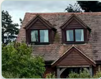
Gable dormers and porch with timber weatherboarding
