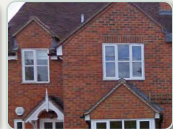
Gable wall dormer and porch aligned to gable front extension
