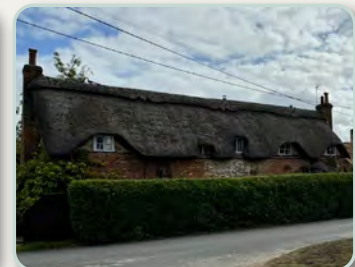
Traditional thatch roof with gable ends and eyebrow dormers
