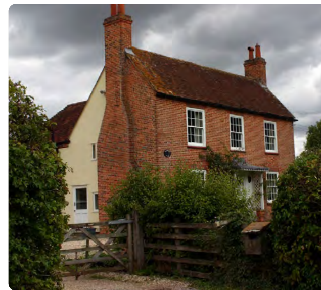
Figure 42: Clapper's Farm, featuring a mix of red brick and cream rendered façade, chimneys on each end of a gable roof and symmetrical sash windows. Copyright: David Kemp
