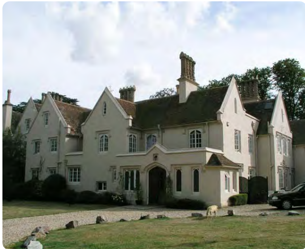
Figure 12: The Grade II listed Silchester House, a mid-19th century tudor style house. Copyright: Andy Potter
