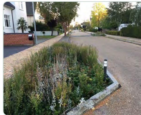
Figure 65: Landscaped areas that narrow the street width for traffic calming that supplements the area's natural atmosphere (taken elsewhere in the UK).
