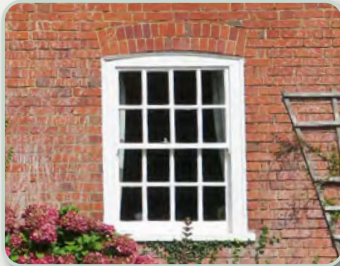
Painted timber sash window with glazing bars and arched brick lintel
