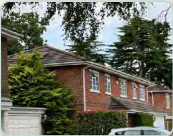
Brown tile hipped roofs with matching hipped roof over garage
