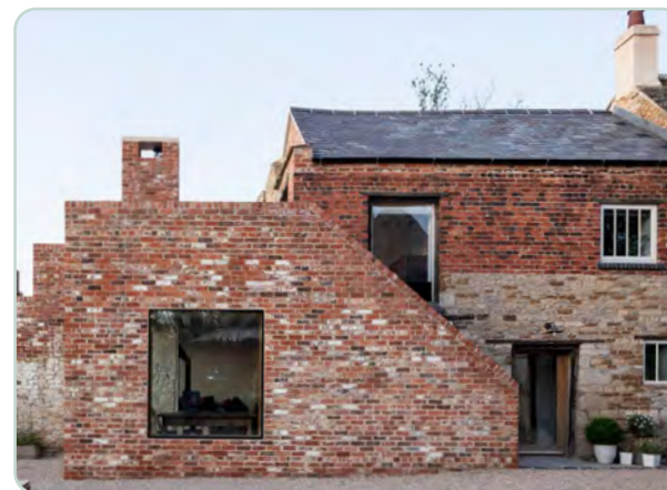
Figure 72: Recycled and reclaimed bricks used for an extension to a traditional dwelling in Gretton, UK. Image credit: Johan Dehlin, Source: https://www.archdaily.com/
