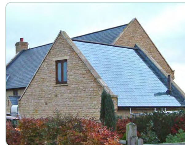
Figure 68: Positive example of implementing solar panels at the start the design stage, resulting in a minimally disrupted building appearance.
