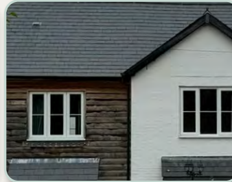
Natural timber weatherboarding, lightly rendered brick
