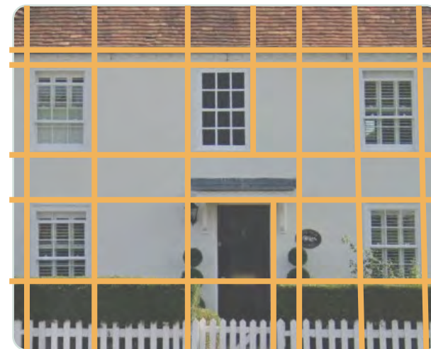
Figure 55: Example of well-proportioned fenestration sizes and placements with consistent material and colour usage.
