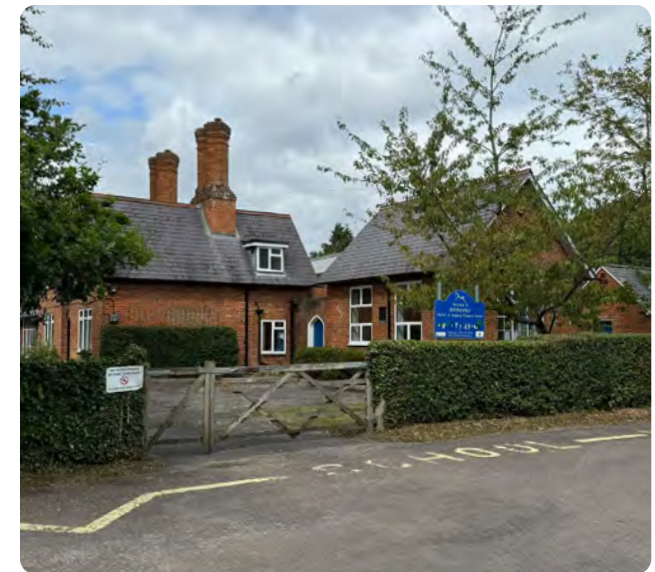
Figure 30: Silchester Primary School uses building materials that reflects those found on other buildings in the village such as slate roof, red brick façades and brick chimney stacks.
