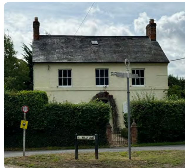
Figure 27: Traditional two-storey house with rendered brick, slate roof, sash windows and boundary directly fronting the road.
