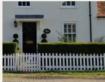
Vertical open panel timber fencing combined with hedgerow
