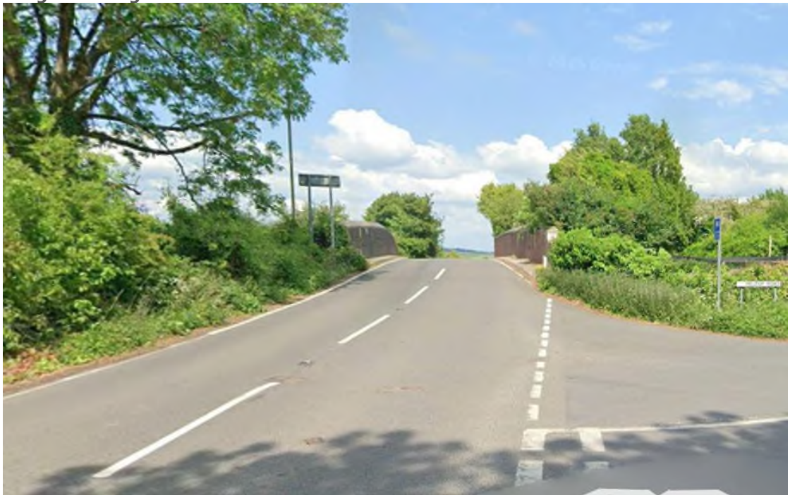
Image 3.6: Kingsclere Road northbound
