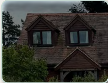
Gable dormers and porch with timber weatherboarding
