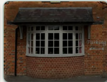
Casement bay window with brick base and tiled roof
