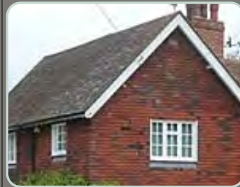
Red and brown hang tiles and painted roof fascias
