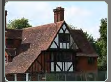
Mock-Tudor half timbering roof structure beams and columns
