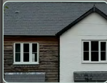
Natural timber weatherboarding, lightly rendered brick
