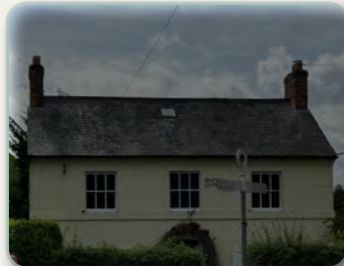
Slate grey gable end roof with red brick stack chimneys
