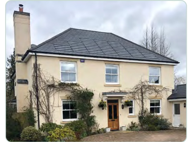
Figure 67: Use of shingle-like solar panels on a slate roof, with the design and colour of the solar panels matching those of the adjacent slate tiles.
