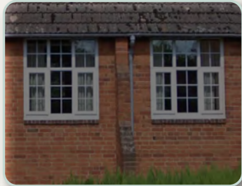
Symmetrical casement windows with narrow brick cills
