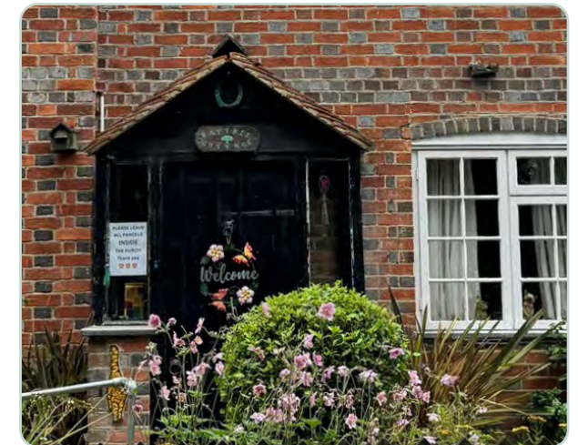
Figure 56: Timber and brick gable roof porch that is aligned to the fenestration to make for a well-proportioned façade.
