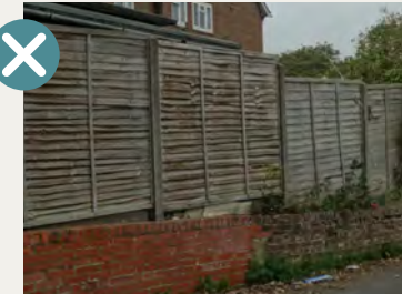
Non-permeable slatted high timber fencing fronting the pavement
