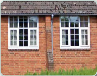
Symmetrical casement windows with narrow brick cills
