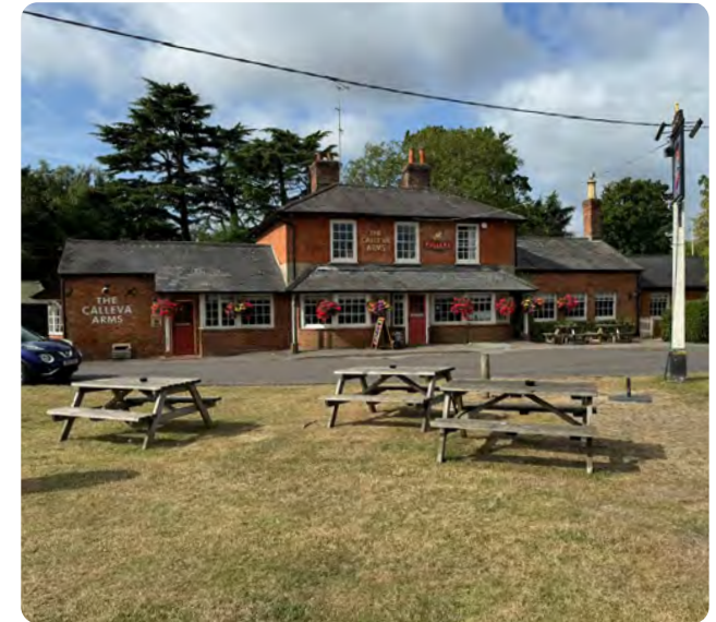
Figure 24: The Calleva Arms features a tiled hipped roof with smaller scaled catslide overhang roofs at the front and defining white frame windows spanning the façade.
