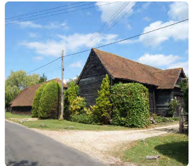
Figure 40: Lower Farm on Bramley Road featuring a dark timber weatherboarding and red tiled roof, with the barn having a dramatic slope and mansard end. Copyright: Des Blenkinsopp
