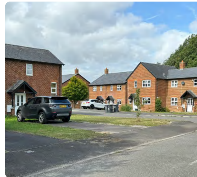
Figure 31: Early Lands cul-de-sac located on the edge of the village boundary is an example of more recent development.
