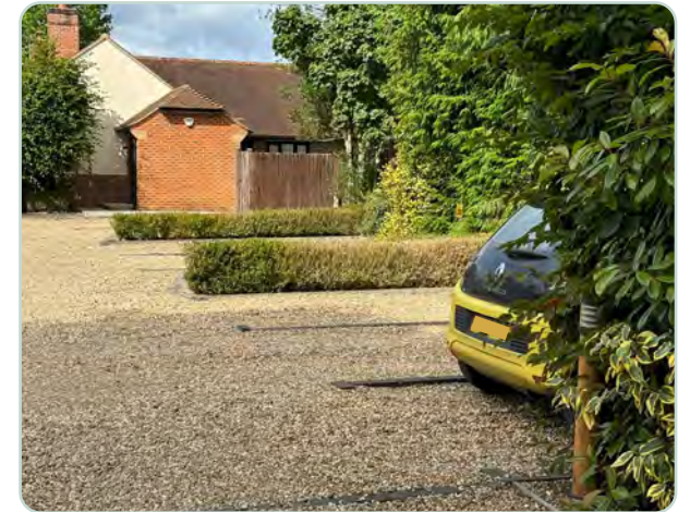
Figure 60: Parking courtyard within the Romans development that has permeable surfacing, natural row dividers and is well overlooked by surrounding dwellings.
