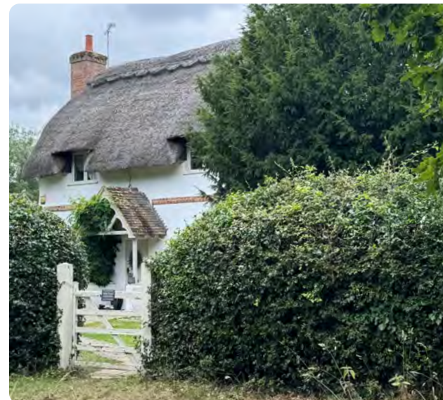
Figure 26: Grade II listed Yew Tree Cottage, early 19th century with thatch roof, eyebrow dormers, rendered façade with row of stacked bond brickwork and a timber gable porch with tiles.
