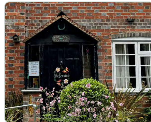
Figure 56: Timber and brick gable roof porch that is aligned to the fenestration to make for a well-proportioned façade.
