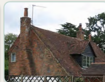
Traditional clay tile catslide roof with larger centred gable dormer
