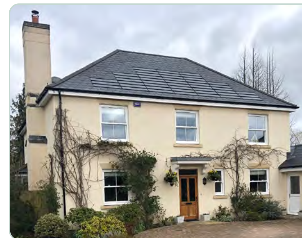
Figure 67: Use of shingle-like solar panels on a slate roof, with the design and colour of the solar panels matching those of the adjacent slate tiles.
