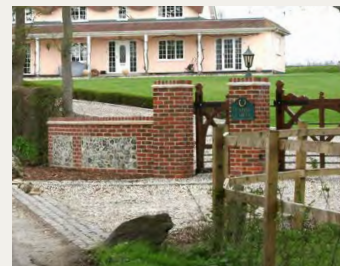
Low brick wall with local stone and a timber entrance gate
