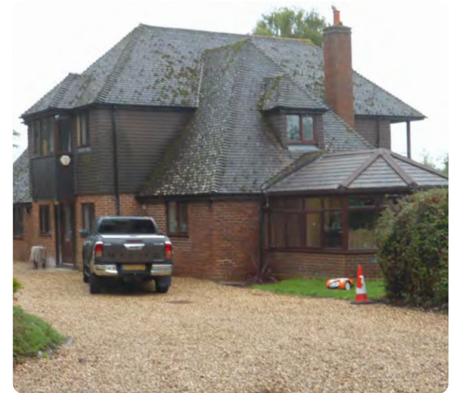
Figure 34: Large dwelling within the Conservation Area that features a distinctive hipped roof and conservatory extension.
